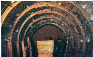
Reconstruction of partly destroyed gallery with steel arches and shotcrete layer.
