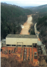
A view of the Peruća HPP power house and switchyard after the explosion. The water was flowing through the destroyed grouting gallery and drainage outlet to the switchyard carrying along the clay core chunks reaching 0.50 m in diameter.
