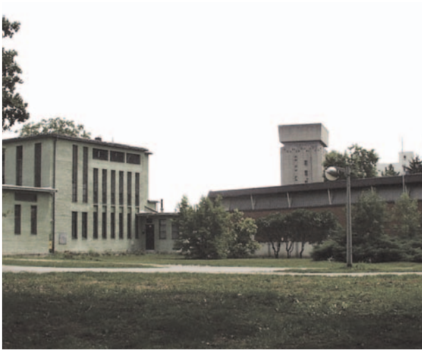
TS 110/35/10 kV Čakovec “Trokut”
