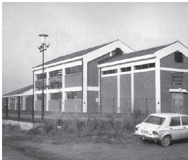
TRANSFORMATORSKA STANICA 35/10 kV VUKOVAR III.
