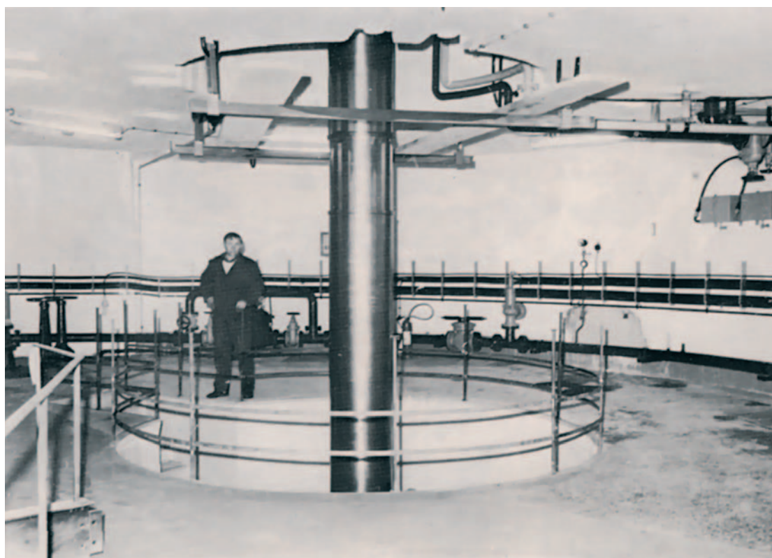
Turbina HE Sklope
