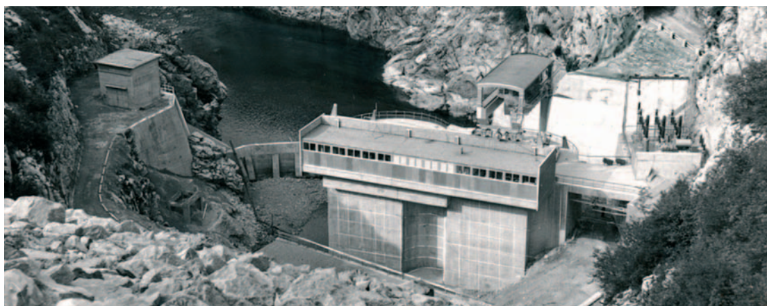
Pogled s brane na strojarnicu HE Sklope
