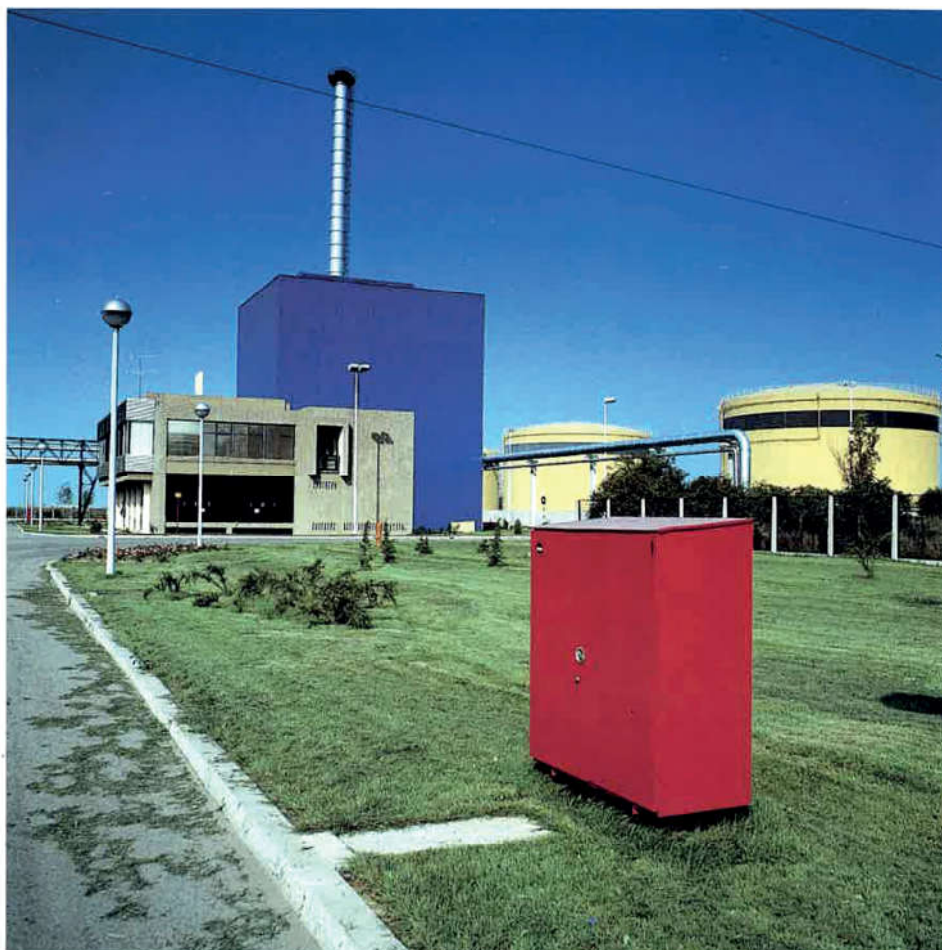
Δ The Osijek combined heat and power plant
