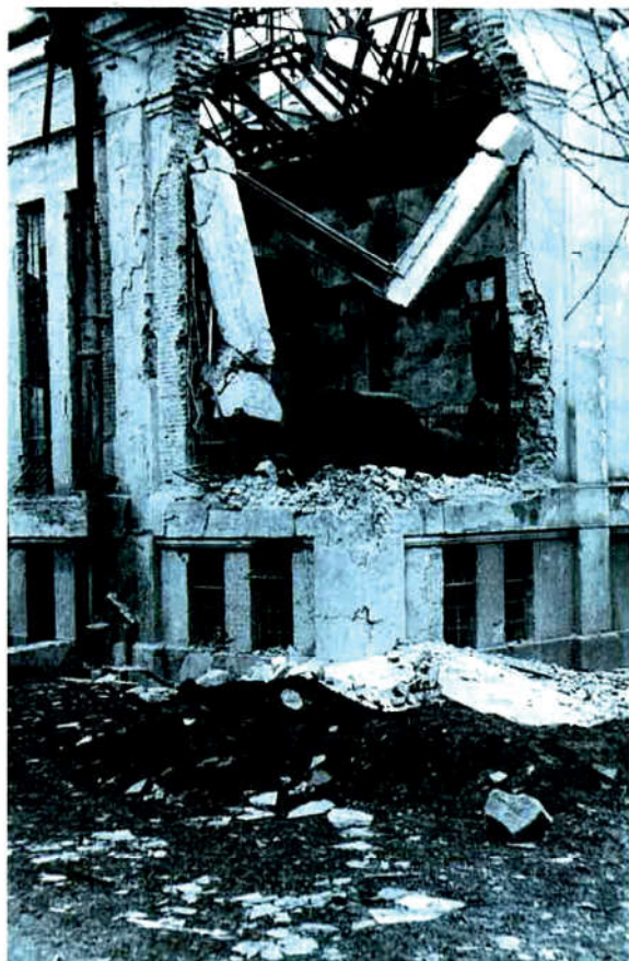
△ War damage to the Osijek power plant, 1944
