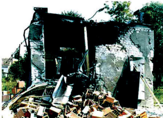
▽ Slavonski Brod - destroyed substation in the Masarikova Street
