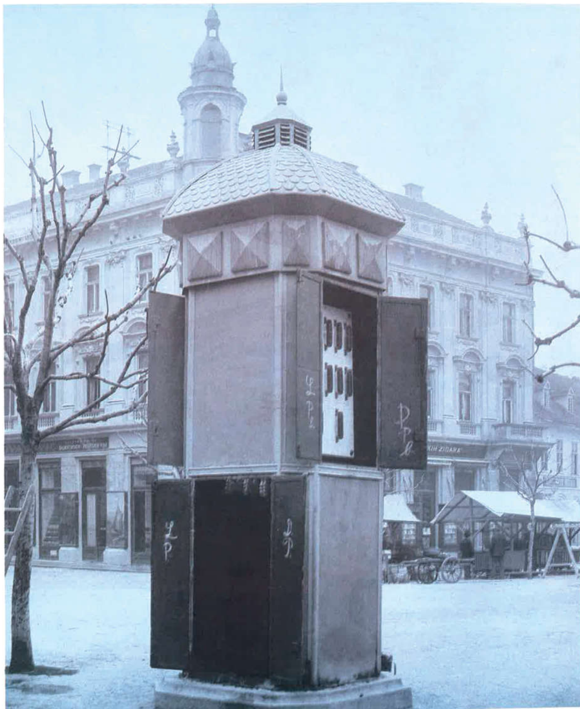
△ An early 5 kV substation in Zagreb
