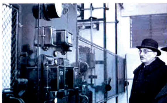
△ A 10 kV substation in Bjelovar
