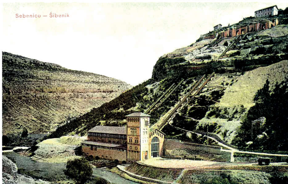
▽ Miljacka (Manojlovac) hydro power plant, constructed 1906
