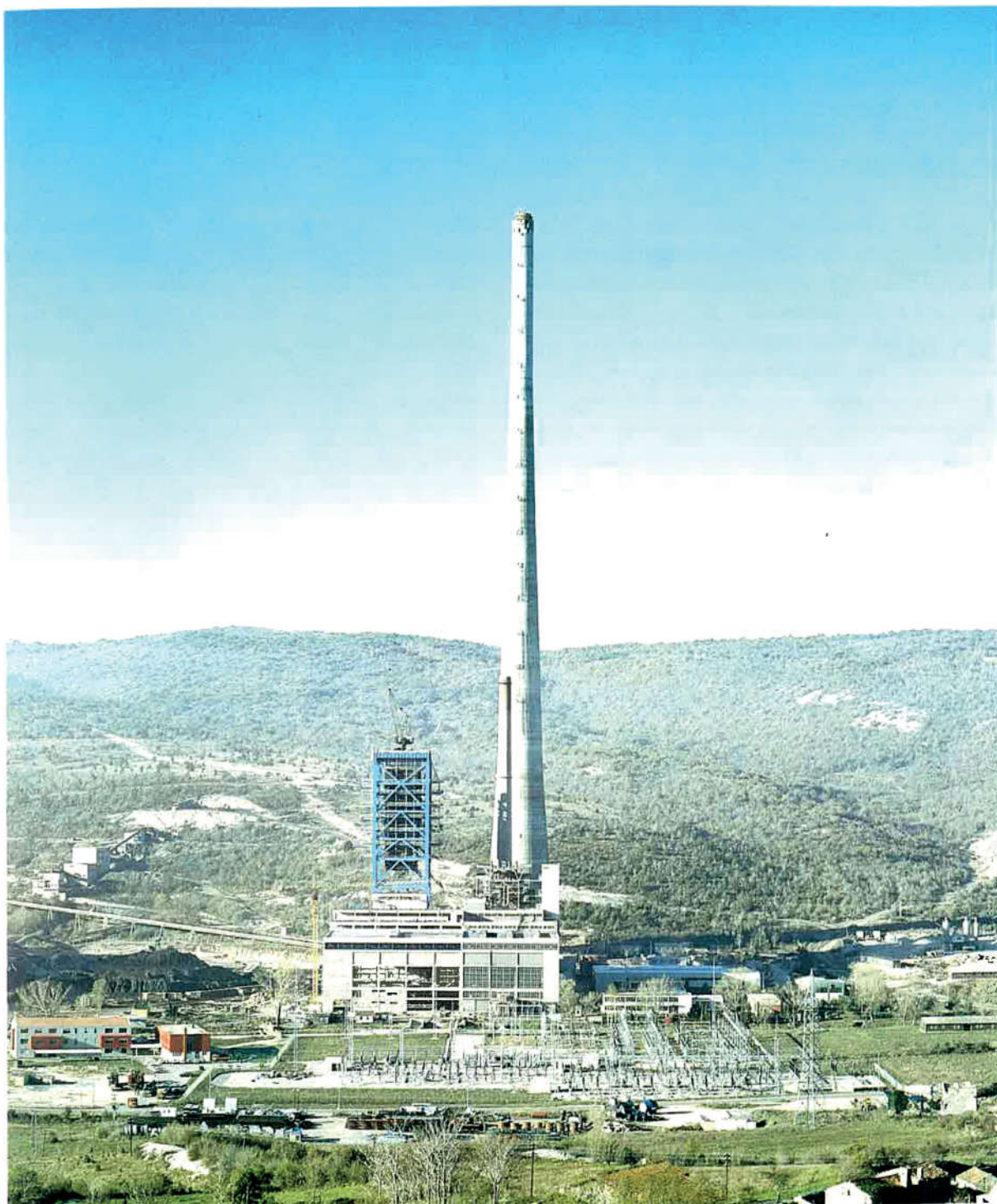
△ The Plomin thermal power plant
