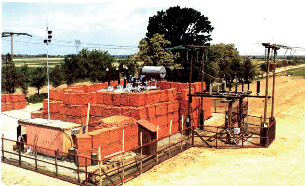
△ Temporary substation built in 1992 after the destruction of the Ernestinovo substation
