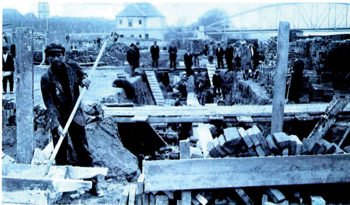
▽ Foundations of the Osijek power plant
