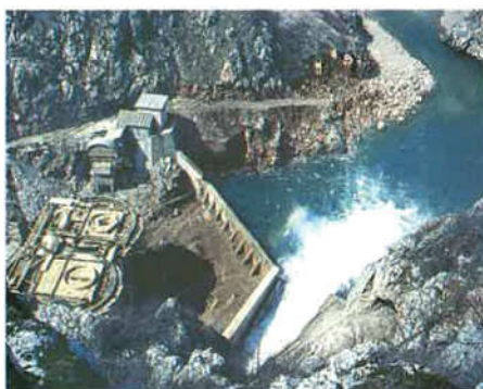
△ Construction of a hydro power plant
