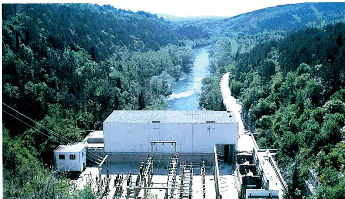
▽ The Peruća hydro power plant
