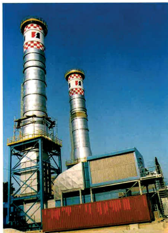
△ Gas fired thermal power plant Dujmovača, Split, 1994
