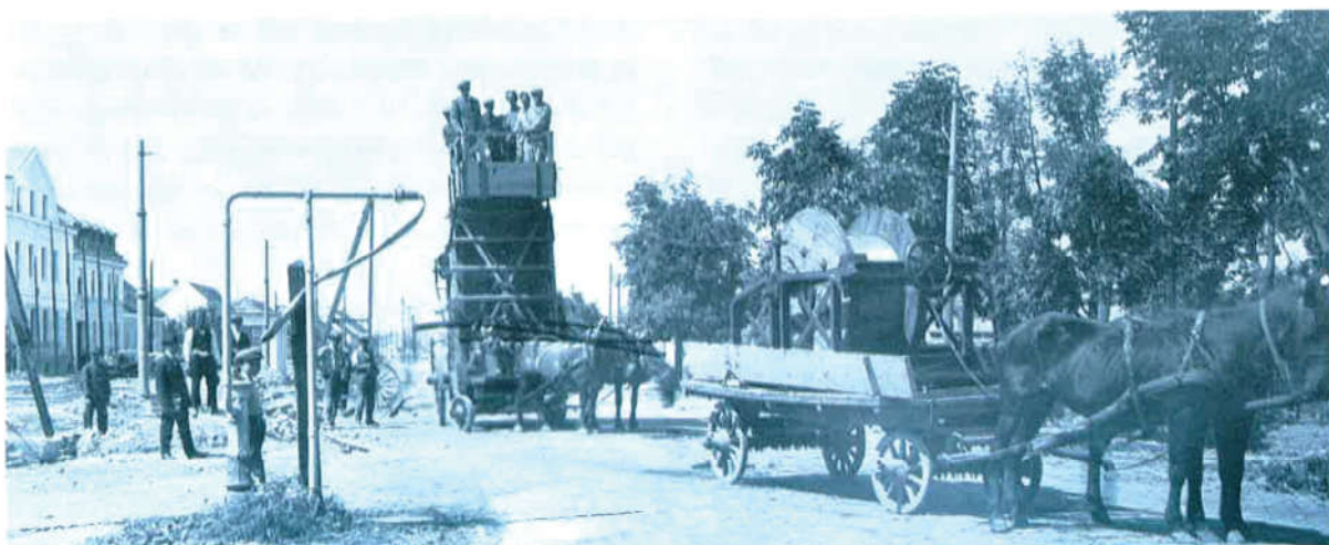
△ Installing streetcar conductors in Osijek
