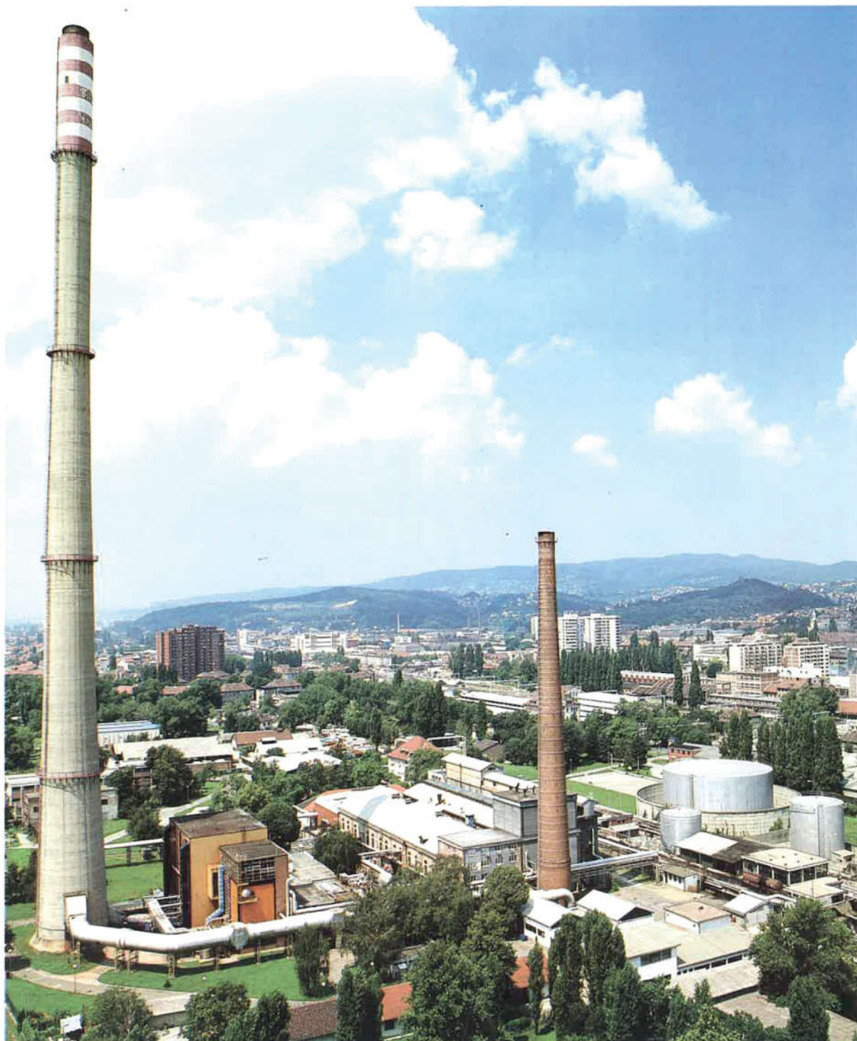
Δ The Zagreb West combined heat and power plant
