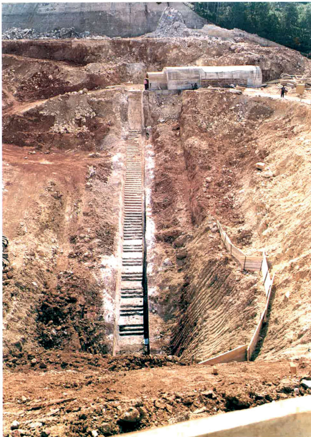
△ Initial remedial works on the Peruća dam
