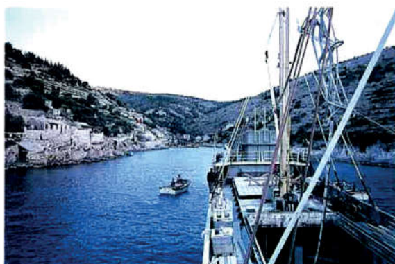
△ Laying of a 110 kV submarine cable
