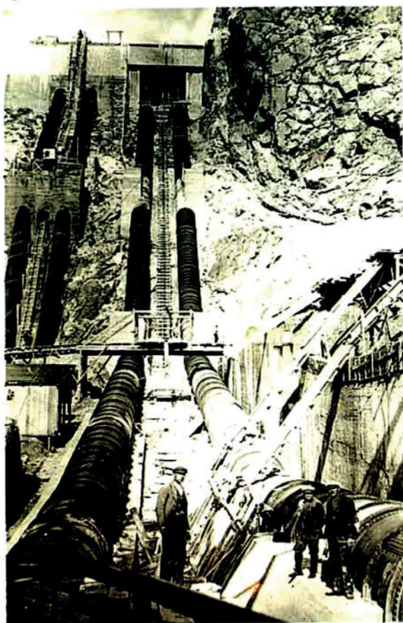
Construction of the Kraljevac hydro power plant
