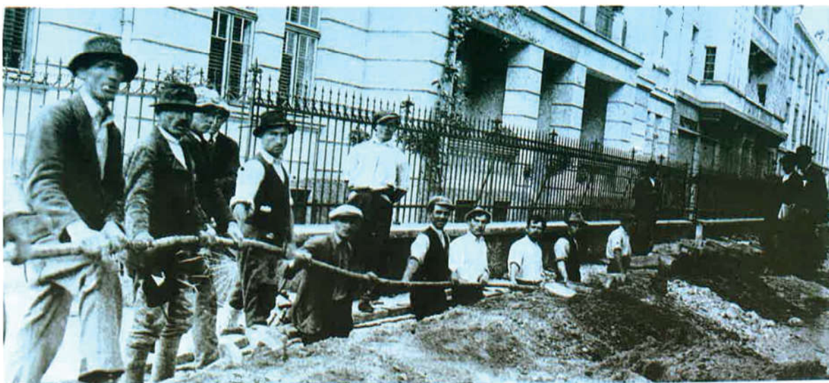
▽ Laying of a 3 kV cable in Osijek, 1926
