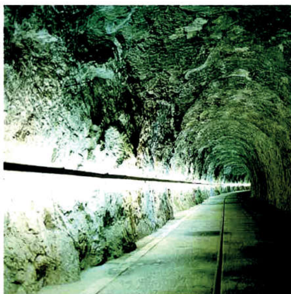
▽ Access tunnel of the hydro power plant
