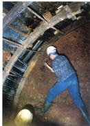
Reconstruction of the completely destroyed gallery; excavation of clayey material mixed with the concrete blocks from the gallery, carried out under the protection of steel arches and concrete panels.
