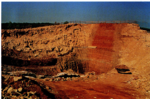
Photo 2. July 2, 1994 - Left dam end - completed excavation
