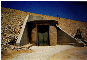
Photo 43. Bottom outlet auxiliary gate house and protective wall
