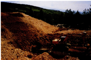
Photo 3. September 15, 1994 - Right dam end - completed excavation
