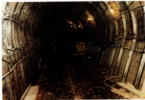
Photo 15. Gallery supported with the steel arches
