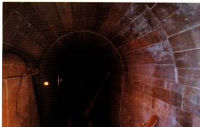
Photo 19. Reconstruction of the completely demolished gallery with 80 cm concrete lining
