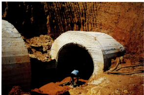
Photo 4. Grouting gallery excavation between the stations 0+90.58 and 0+93.00 from July 12 to July 28, 1994, through the uncreted part of the gallery
