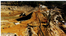
PERUĆA HYDROELECTRIC POWER PLANT
