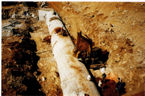
Photo 35. August 12, 1994 Beginning of the material building in into the right dam end
