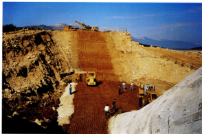
Photo 34. September 7, 1994 Building in of the material into the left dam end, El. 338.50 m a.s.l.
