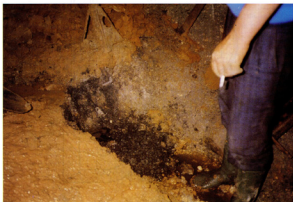
Photo 23. Burned concrete
