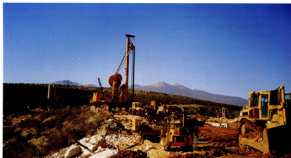
Photo 45. December 2, 1994 Plastic concrete cut-off wall construction and building in of material in the left dam end
