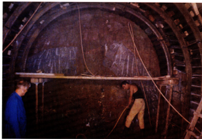
Photo 17. Supporting the excavation site with steel arches and plates - the caved-in concrete blocks are visible
