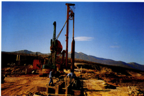
Photo 44. December 16, 1994 Completion of guide walls and panel excavation by hydraulic trench cutter - left dam end
