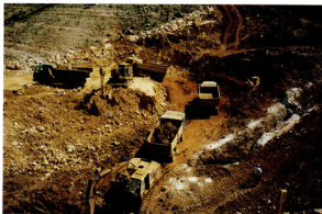
Photo 25. Excavation in the left dam end - Traffic on the upstream ramp
