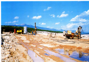
Photo 49. Grouting from the El. 353.00 m a.s.l
