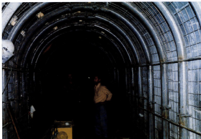
Photo 13. Onset of the grouting gallery reconstruction works
