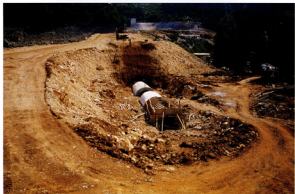
Photo 22. July 21, 1994 Grouting gallery works in the right dam end
