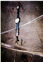
Photo 10. Grouting gallery convergence measurement
