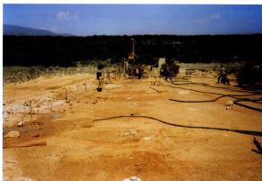
Photo 3. Clay core grouting
