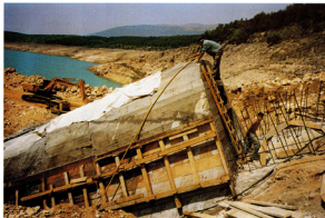
Photo 29. Grouting gallery reconstruction in the left dam end
