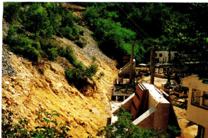
Photo 41. August 2, 1994 Downstream dam toe retaining wall during construction
