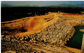
Photo 2. Left dam end excavation completed
