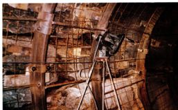
Photo 4. Gallery reconstruction with steel arches, shotcrete and grouting - detail
