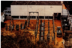
Photo 1. January 29, 1993 - Switchyard drainage shaft
