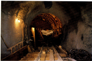
Photo 20. October 19, 1994 Preparation of formwork for placement of concrete between the stations 1+17.53 and 1+22.78
