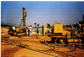
Photo 2. Clay core grouting
