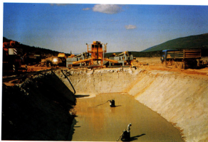
Photo 2. Slurry desanding plant BE 500 with the trench slurry tank
