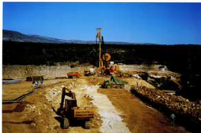
Photo 39. September 23, 1994 Building in the right dam end filter; El. 353.20 m a.s.l.
