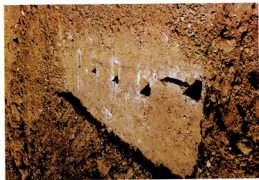
Photo 7. Pits dug in a clay core for placement of cells in different directions
