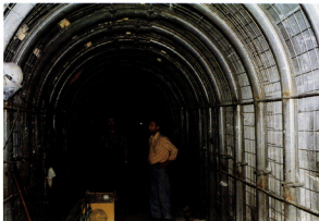
Photo 8. Access tunnel No. 2 after placement of steel arches
