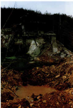
Photo 4. Left dam end and spillway
