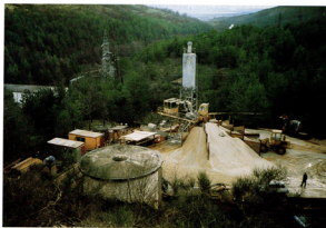
Photo 16. Grouting gallery reconstruction site facilities
