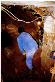
Photo 19. September 21, 1994 Gallery drainage pipe excavation in station 1+42.00
