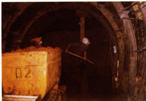
Photo 21. Loading excavated material on rail vans
