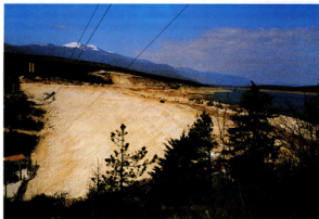
Photo 1. Final dam remediation works
