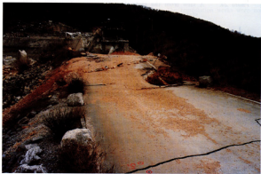
Photo 23. Crater between the stations 0+82.00 and 0+89.00
