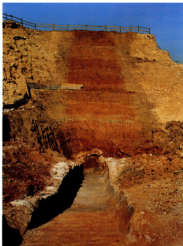
Photo 14. July 2, 1994 Left dam end and grouting gallery
