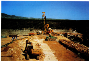
Photo 5. Backfilling downstream filter trench
