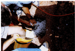
Photo 5. Pore-water pressure cell placement into the dam clay core
