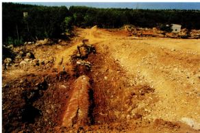
Photo 24. Partly demolished gallery in the right dam end
