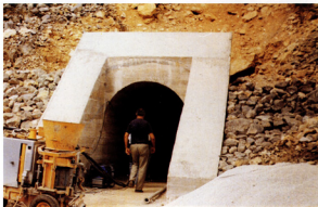
Photo 7. Reconstructed access tunnel No. 2 portal
