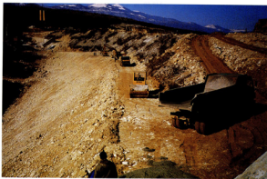
Photo 37. March 10, 1995 Building in of the material into the downstream shell; dam widening for 5.0 m; El. 345.00 m a.s.l.
