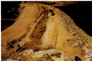
Photo 7. Dam body construction works above the El. 353.00 and 358.00 m a.s.l
