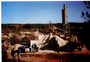
Photo 4. Concrete mixing plant for the gallery remediation, operating platform in front of the access tunnel No. 2
