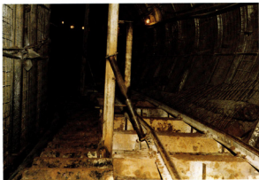
Photo 3. Van rail in the gallery
