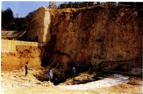
Photo 2. Spillway construction pit and placement of cylinder shaft reinforcement
