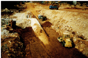
Photo 38. September 1, 1994 Clay building in into the right dam end; El. 348.50 m a.s.l.
