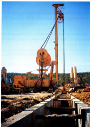
Photo 4. Cut-off wall trench excavation by hydraulic trench cutter
