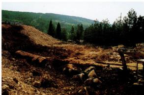
Photo 29. July 2, 1994 Right dam end - removal of damaged gallery sections
