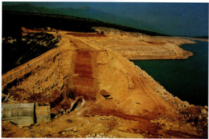
Photo 31. July 1, 1994 Left dam end - completely finished excavation
