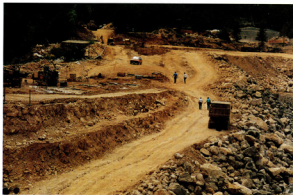
Photo 26. Access ramp towards the left dam end
