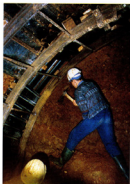
Photo 19. Reconstruction of the completely demolished gallery with 80 cm concrete lining
