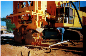
Photo 5. Hydraulic trench cutter wheels
