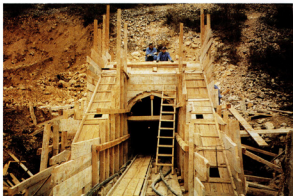
Photo 6. Reconstruction of the access tunnel No. 2 portal
