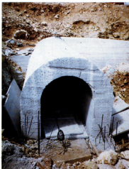
Photo 24. Partly demolished gallery in the right dam end
