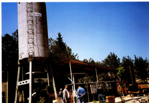
Photo 48. Main grouting post
