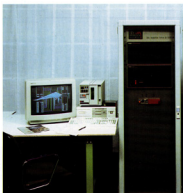
Photo 12. Data Acquisition System
