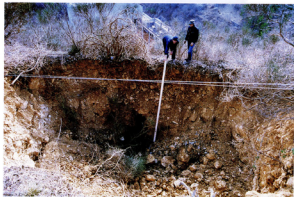
Photo 10. February 16, 1993. - Crater on station 1+52.16 to 1+62.62 - Downward view
