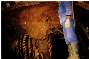
Photo 34. The deepest part of the gallery in the central part
