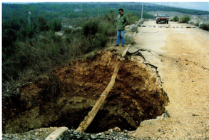
Photo 11. Cavern on station 0+82 to 0+89
