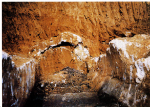
Photo 1. Clay core at the deepest excavated part of the left dam end with destroyed gallery
