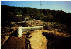
Photo 30. Partly reconstructed gallery
