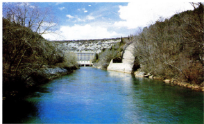
Photo 1. Hydroelectric power plant and dam - downstream view
