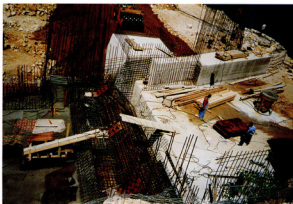
Photo 8. June 21, 1995 - Spillway activities
