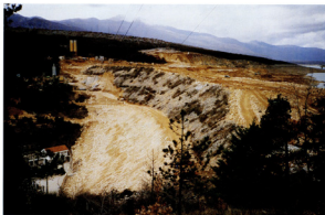
Photo 40. February 27, 1995 Building in of rock material into the downstream shell; El. 339.50 m a.s.l.
