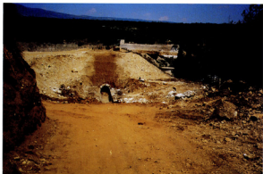
Photo 30. July 15, 1994 Right dam end - completely finished excavation
