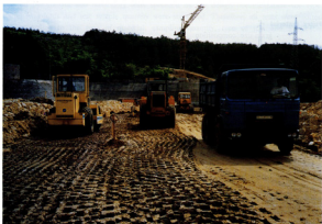
Photo 4. Clay core compacting
