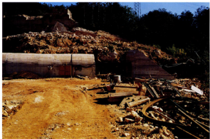
Photo 21. October 11, 1994 Access tunnel to the grouting gallery in the left dam end
