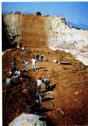
Photo 3. Placement of pore-water pressure cells and total pressure cells in the left dam end
