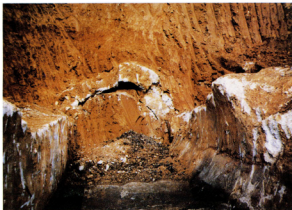
Photo 26. Demolished gallery in the left dam end
