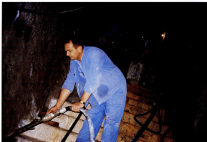
Photo 46. Contact grouting in the grouting gallery
