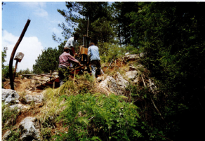
Photo 47. June 19, 1995 Left dam end grouting works
