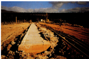
Photo 6. Top of the constructed cut-off wall in the right dam end
