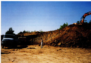
Photo 1. Clay excavation at the Zorica deposit
