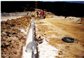
Photo 9. Installation of extensometers into the dam crest
