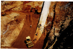
Photo 36. August 19, 1994 Backfilling the left dam end, El. 334.10 m a.s.l.
