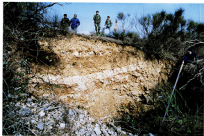
Photo 9. February 16, 1993. - Crater on station 1+12.16 to 1+62.61 - Upward view
