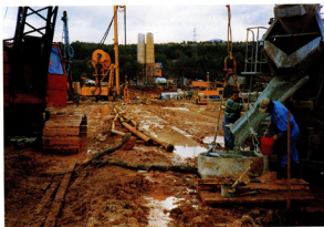
Photo 3. Panel concreting
