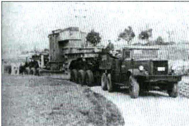
Transport transformatora u TS 110/35 kV Meterize 1955. godine
