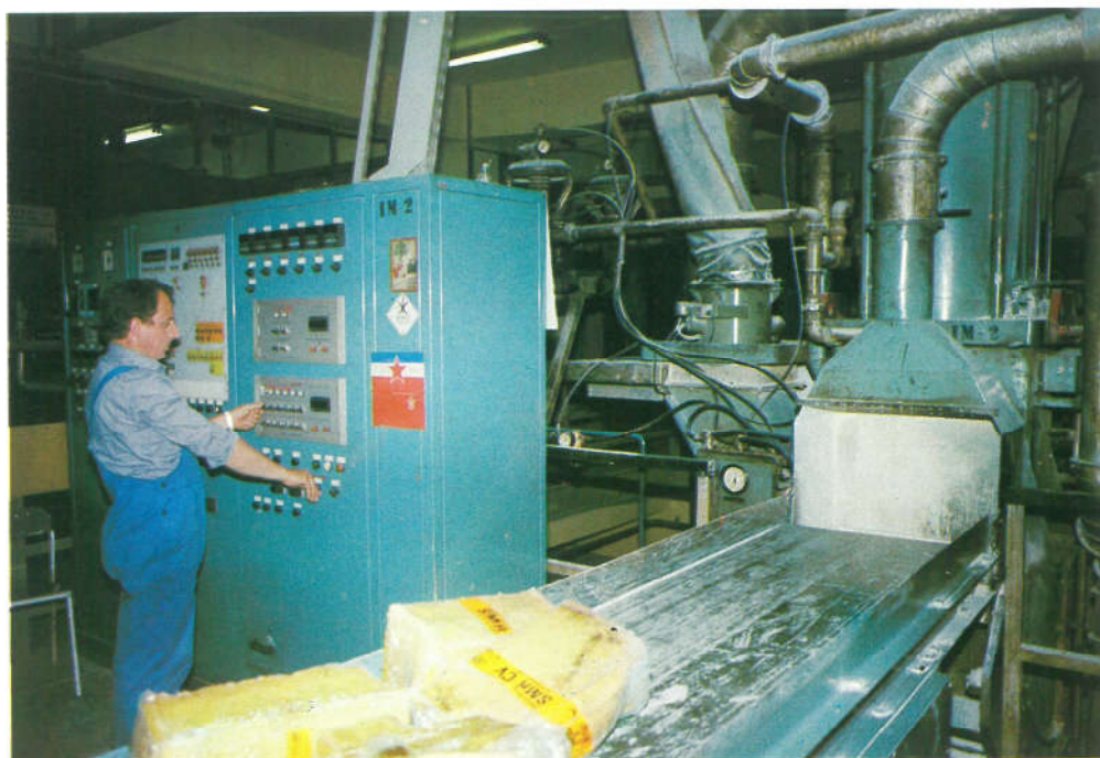
Control panel for rubber compaund mixer
