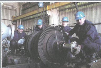
Generalni remont parne turbine
