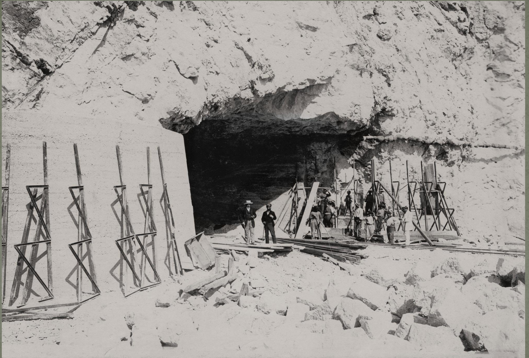
Right outlet from the tunnel to the surge chamber
