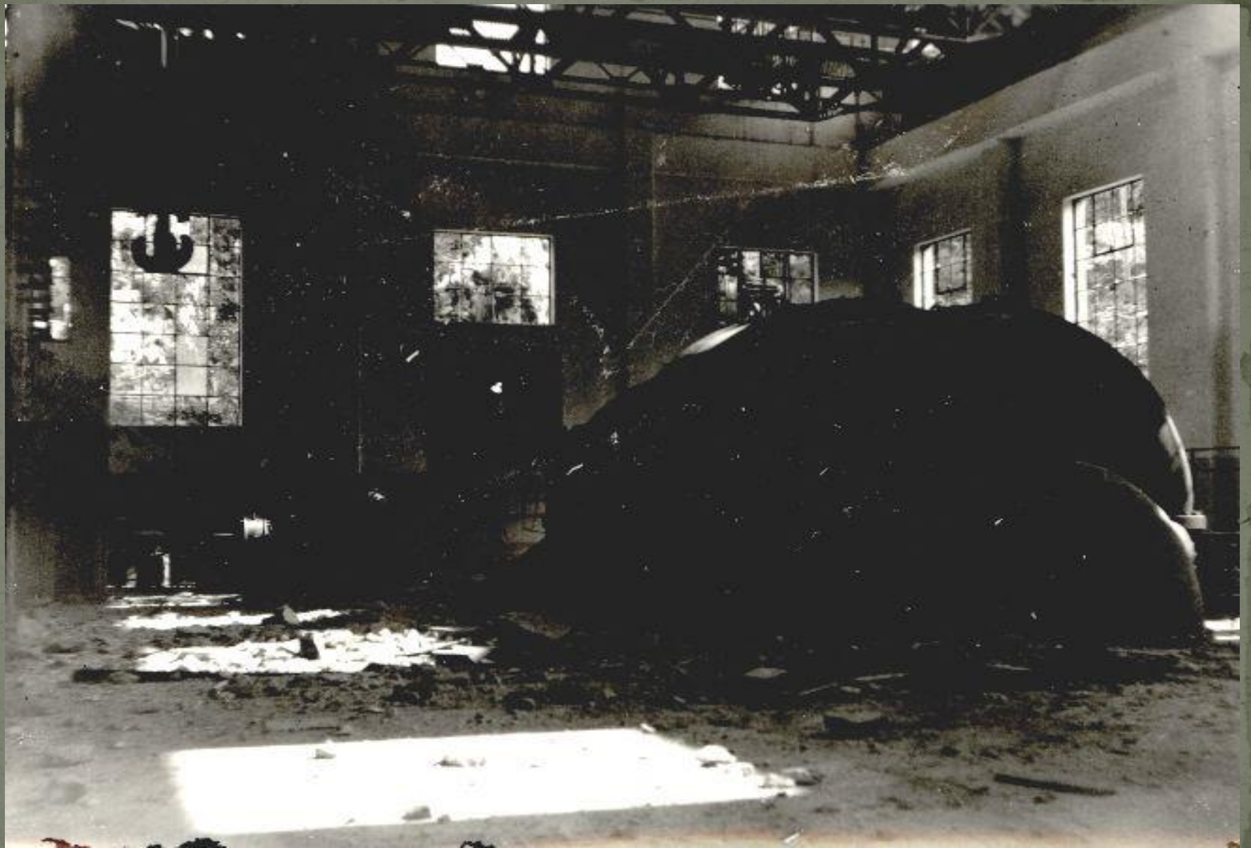
Bombarding of the powerhouse in 1944
