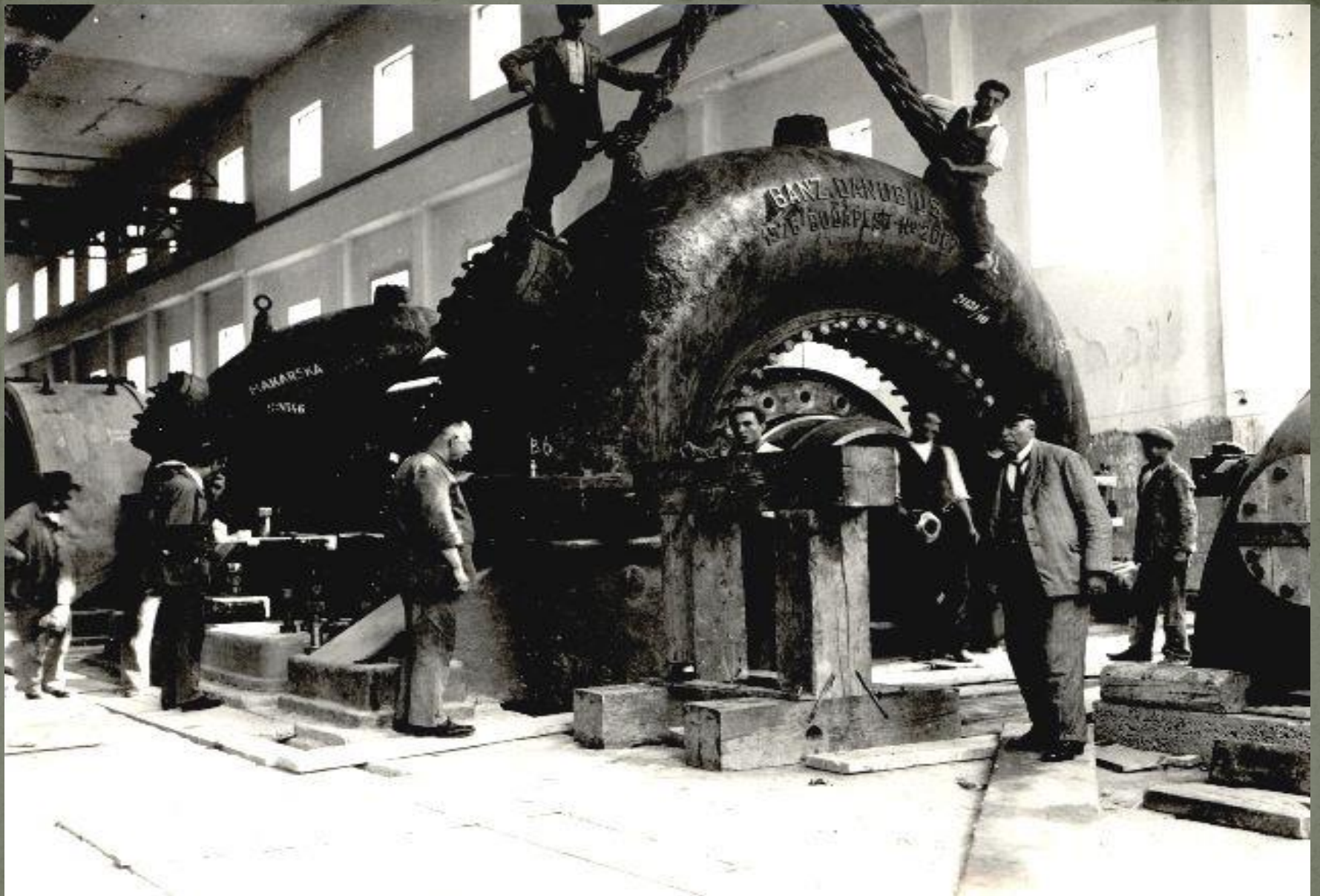
Final works on the erection of the turbine
