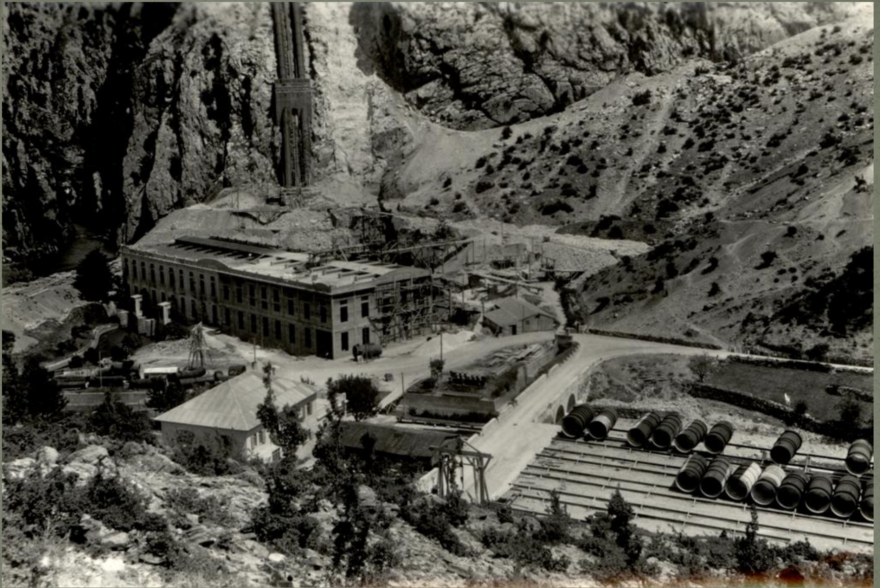
Disposal of the penstock parts in Kraljevac HPP
