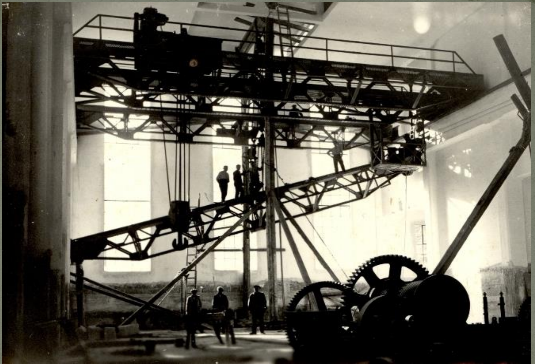
Erection of the bridge crane
