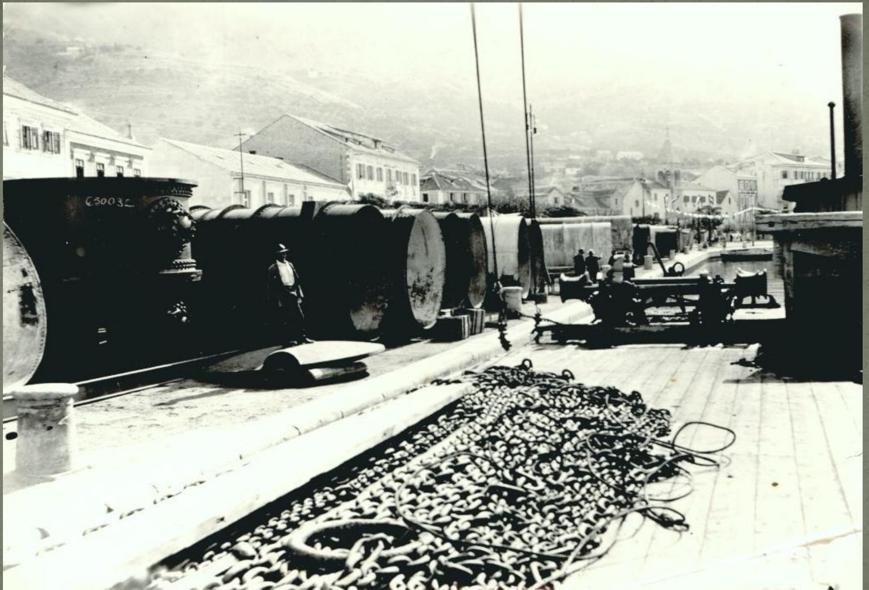
Parts of the penstocks in the Makarska harbour
