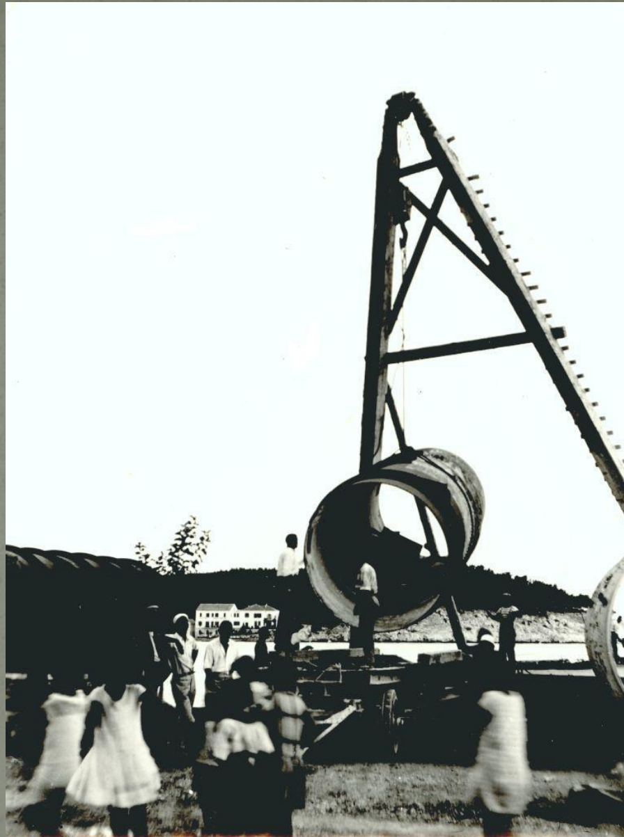
Unloading of the penstocks in Makarska
