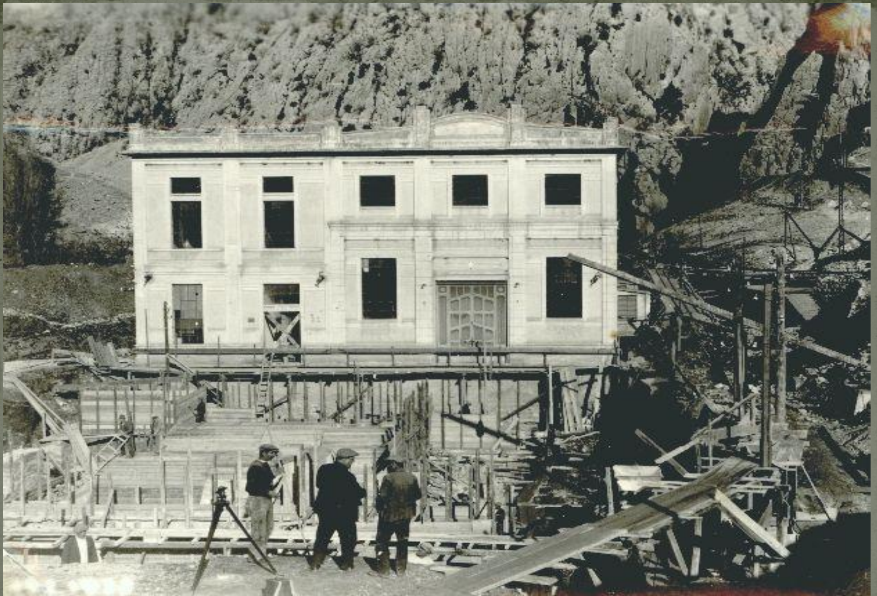
Works on widening the powerhouse
