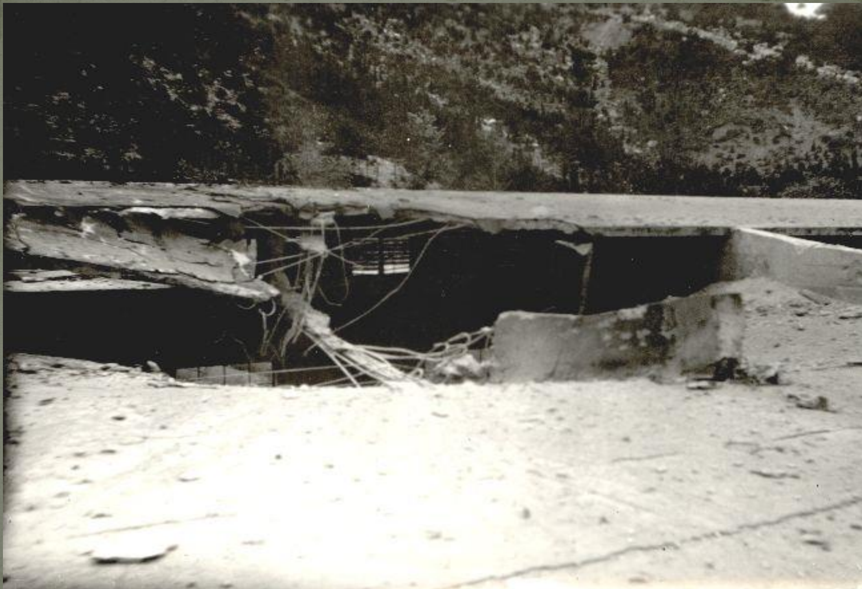
Bombarding of the powerhouse in 1944
