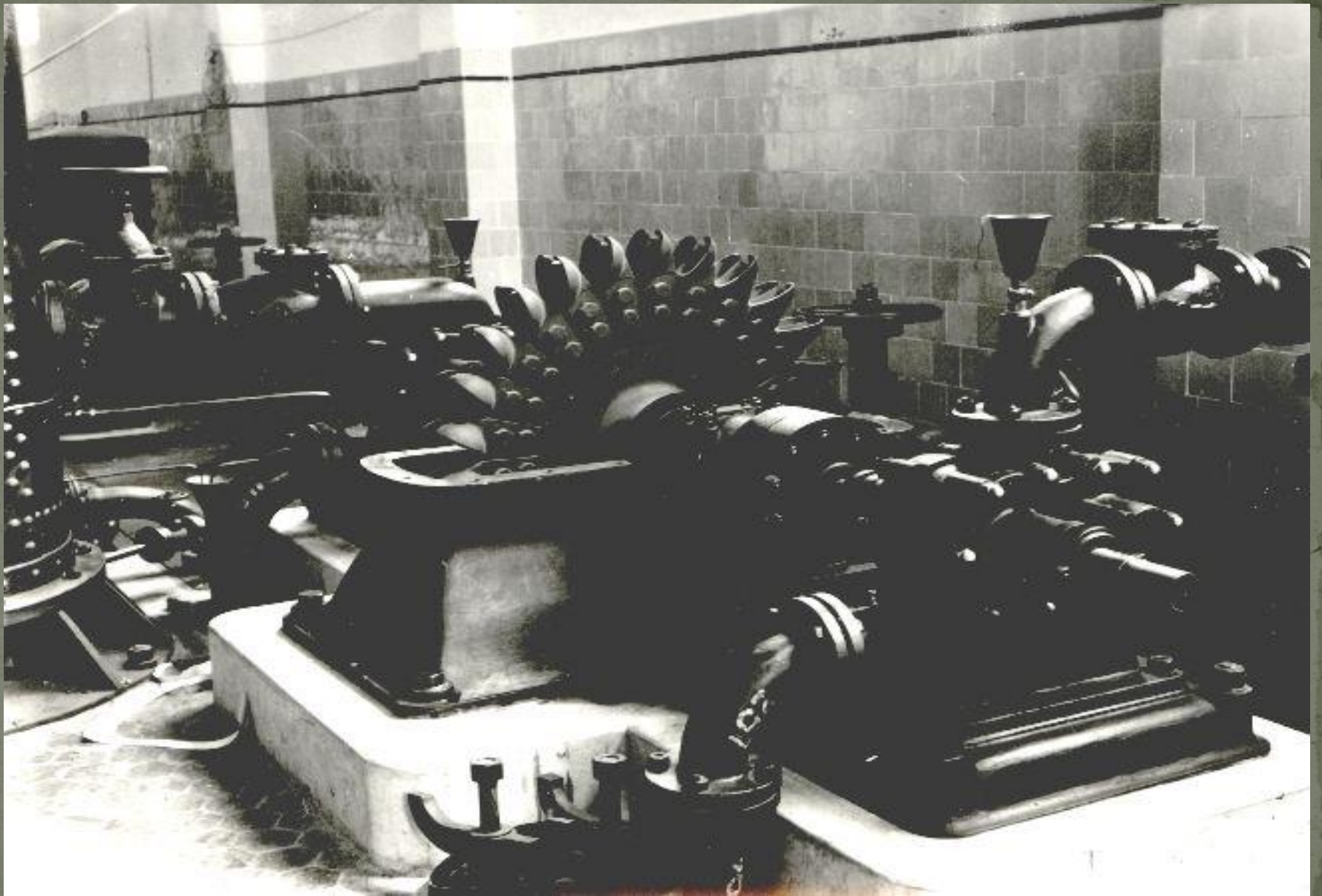
Generating unit auxiliary equipment – Pelton turbine
