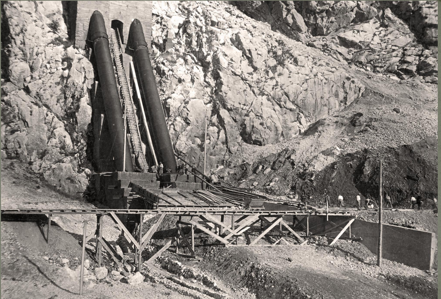
Works on the construction of the first two penstocks
