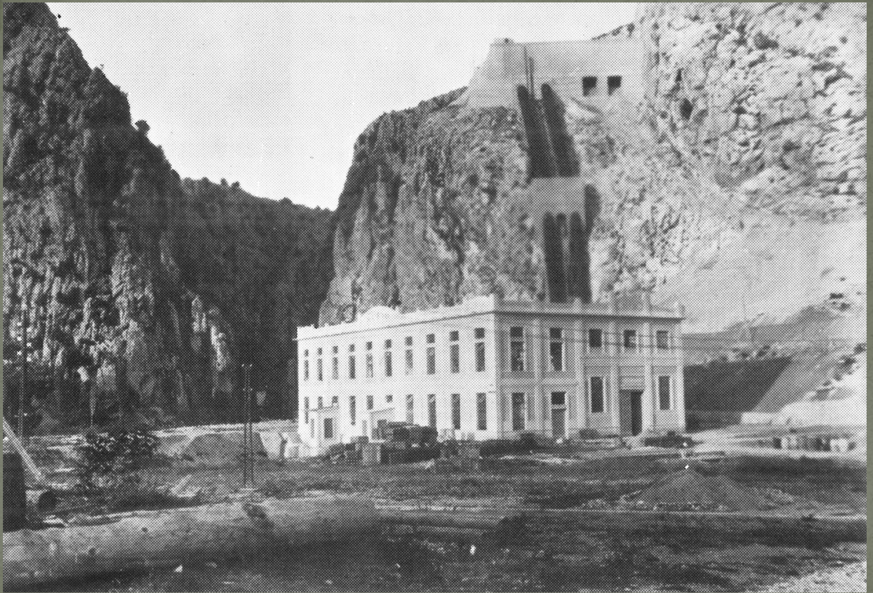
Completed works of the first construction stage
