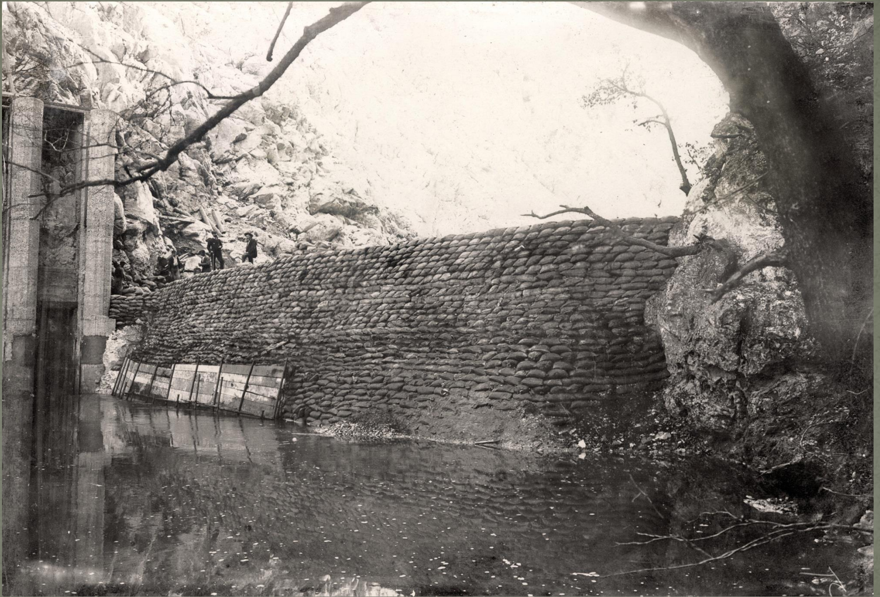
Provisional dam built of 20 000 bags with sand
