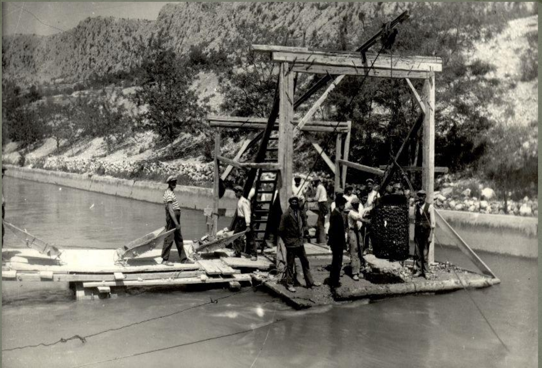
Works in the tailrace canal
