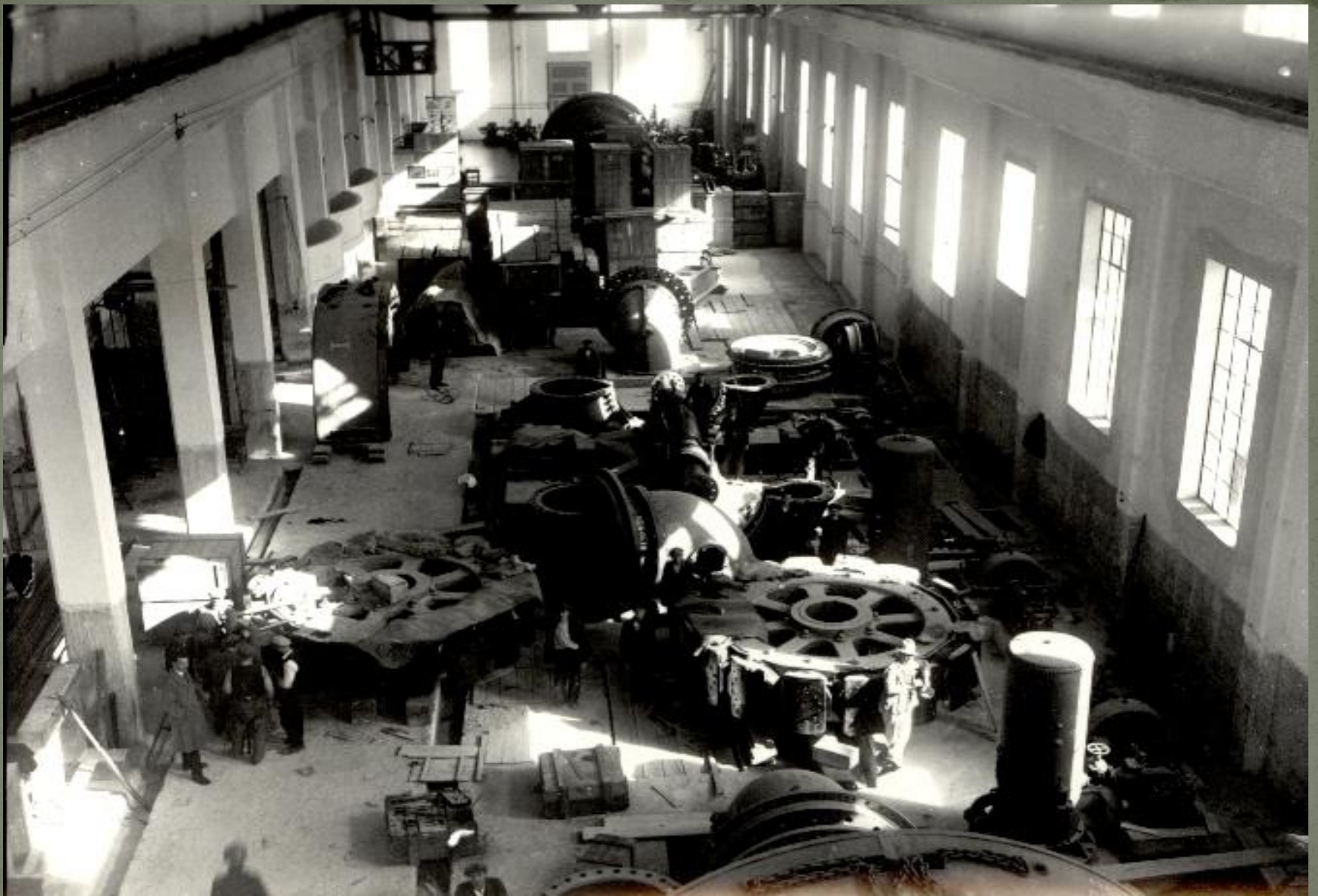
View of the powerhouse
