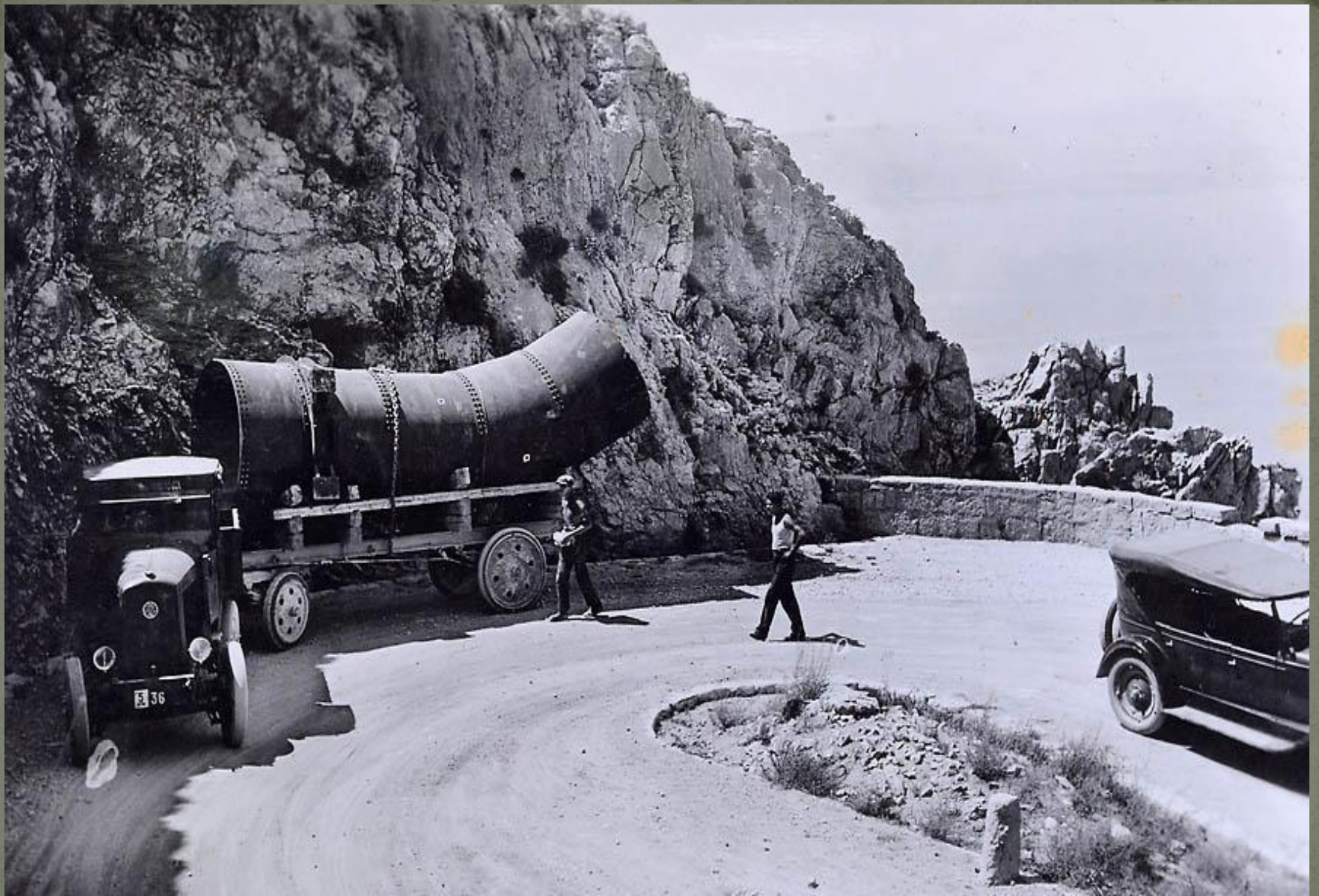
Transportation of the penstocks Makarska - Kraljevac
