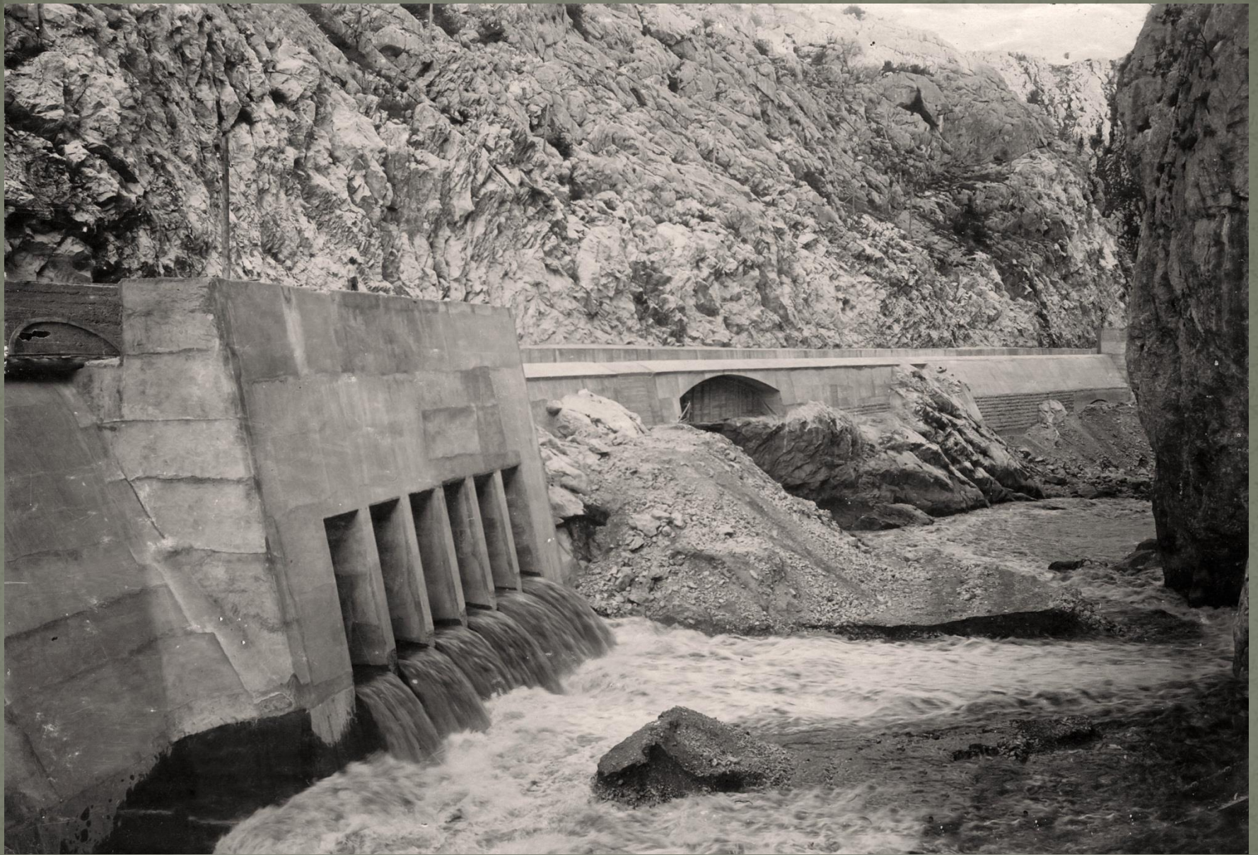
The dam was built – the end of 1911
