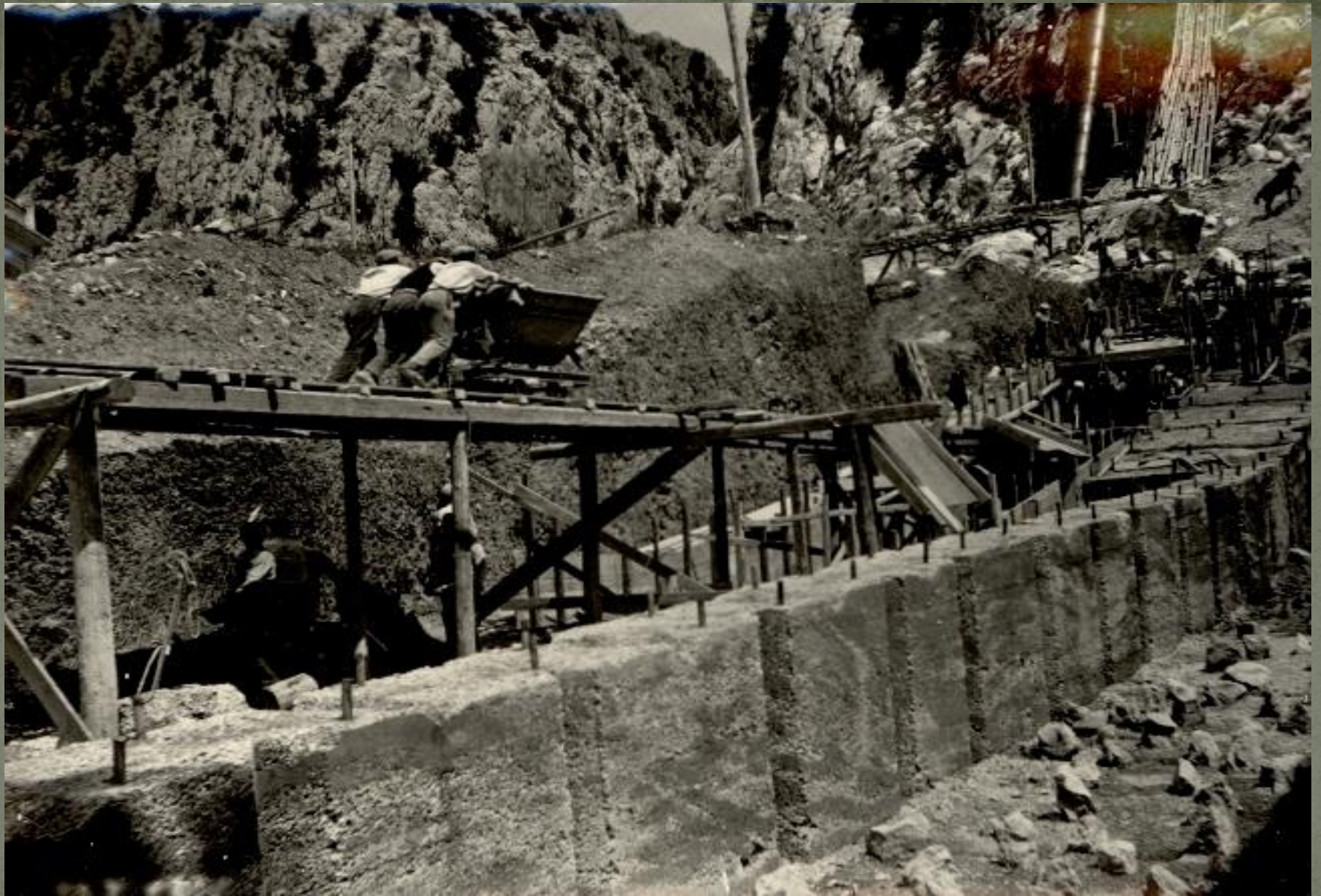
Works on construction of the penstocks 3 and 4
