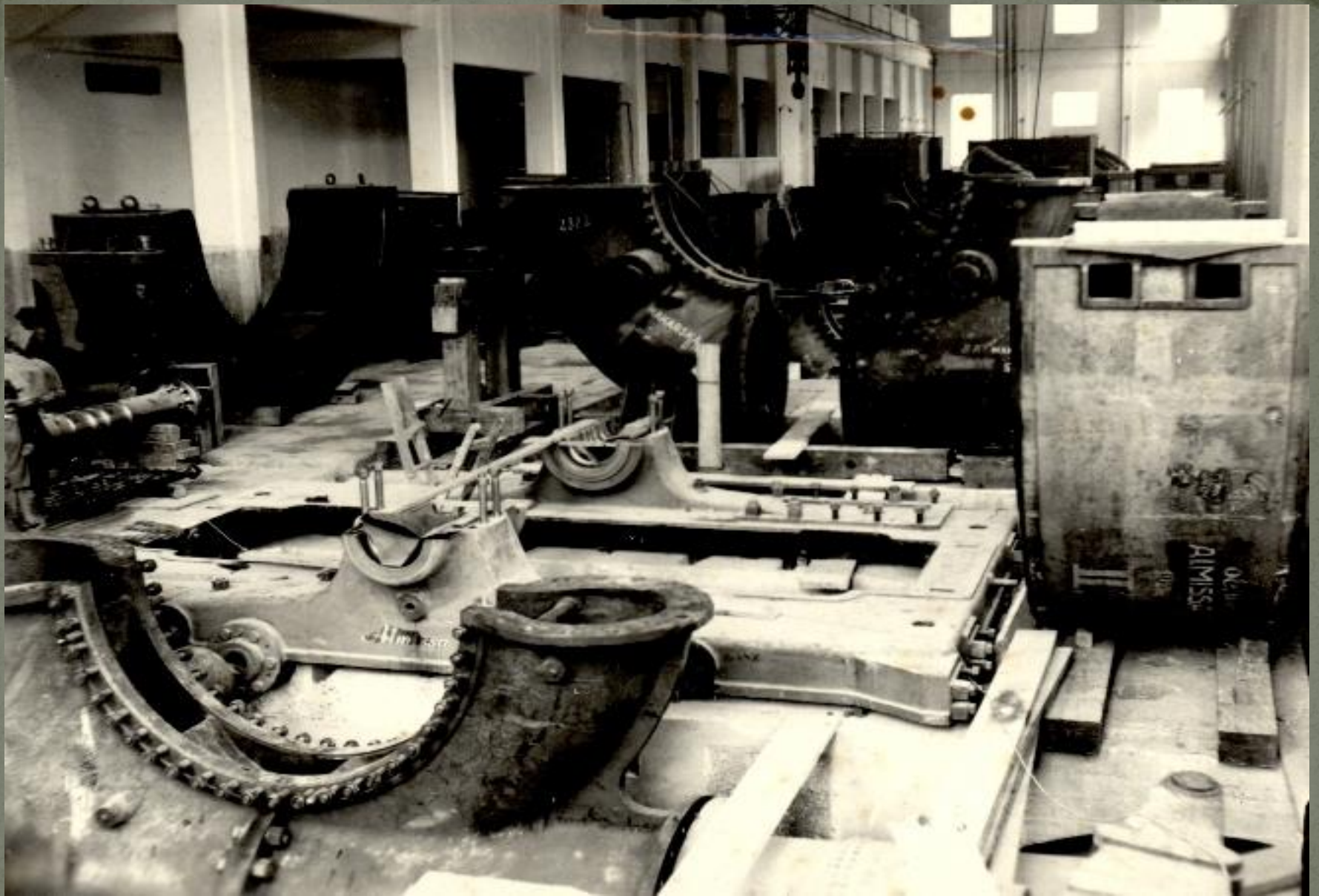
Commencement of the erection works on generating units
