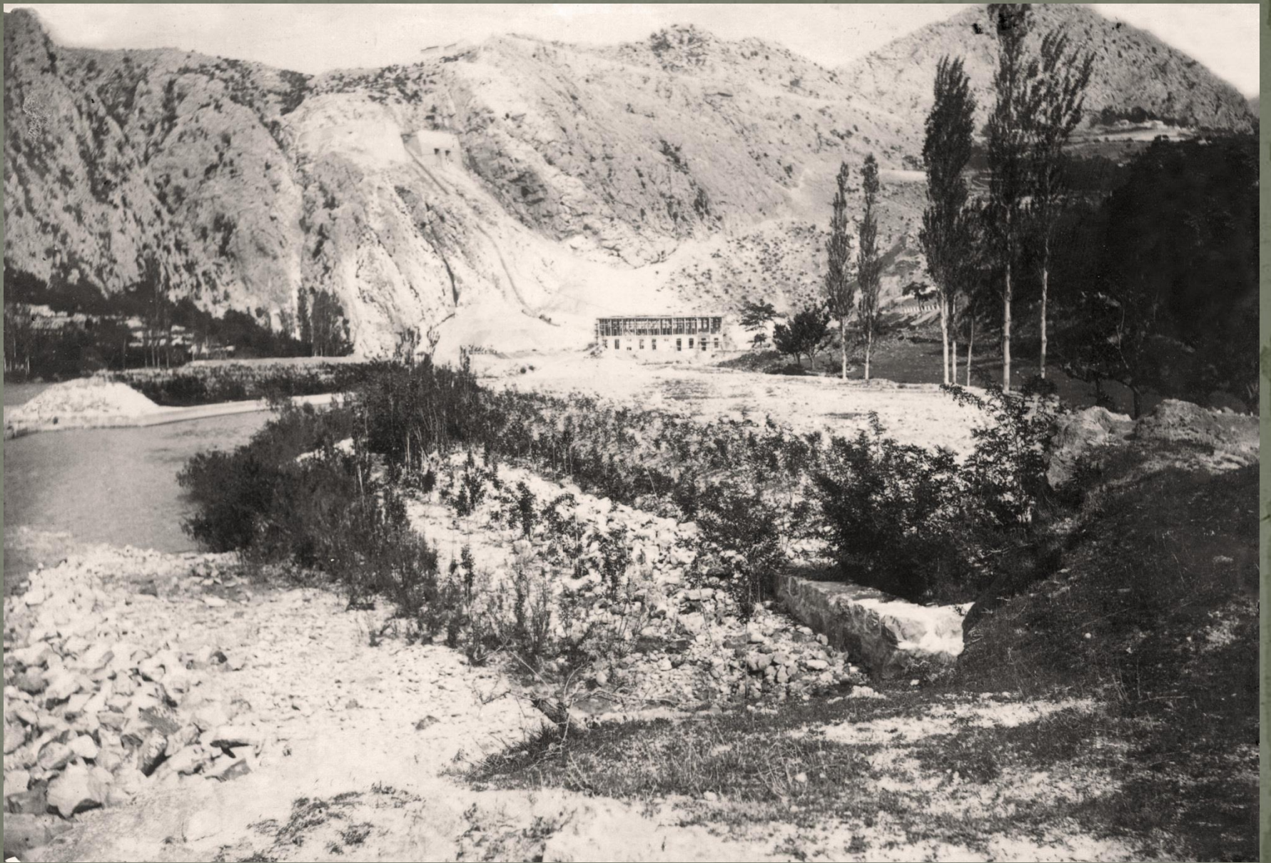
Final construction works of the first stage
