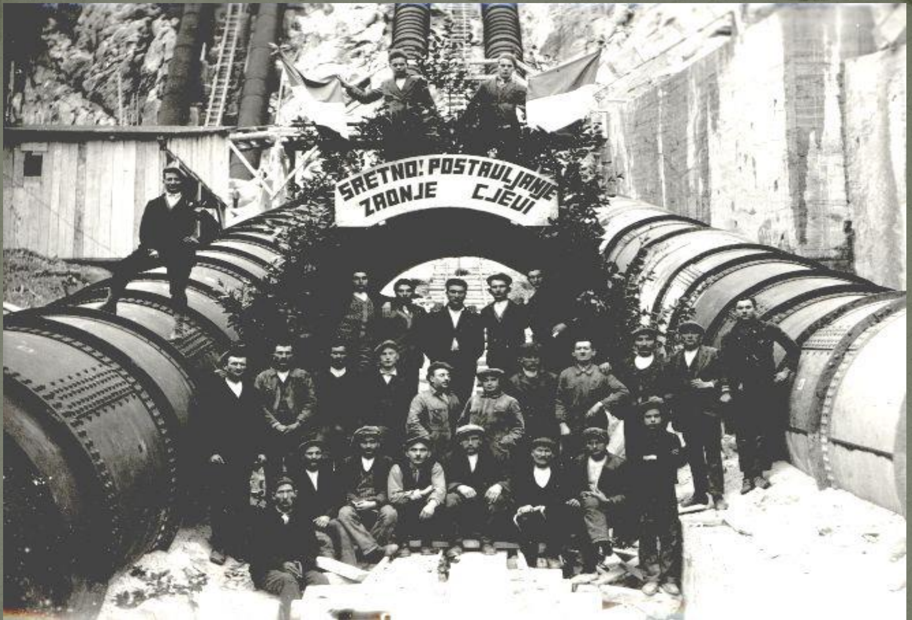
End of the construction works on the penstocks 3 and 4
