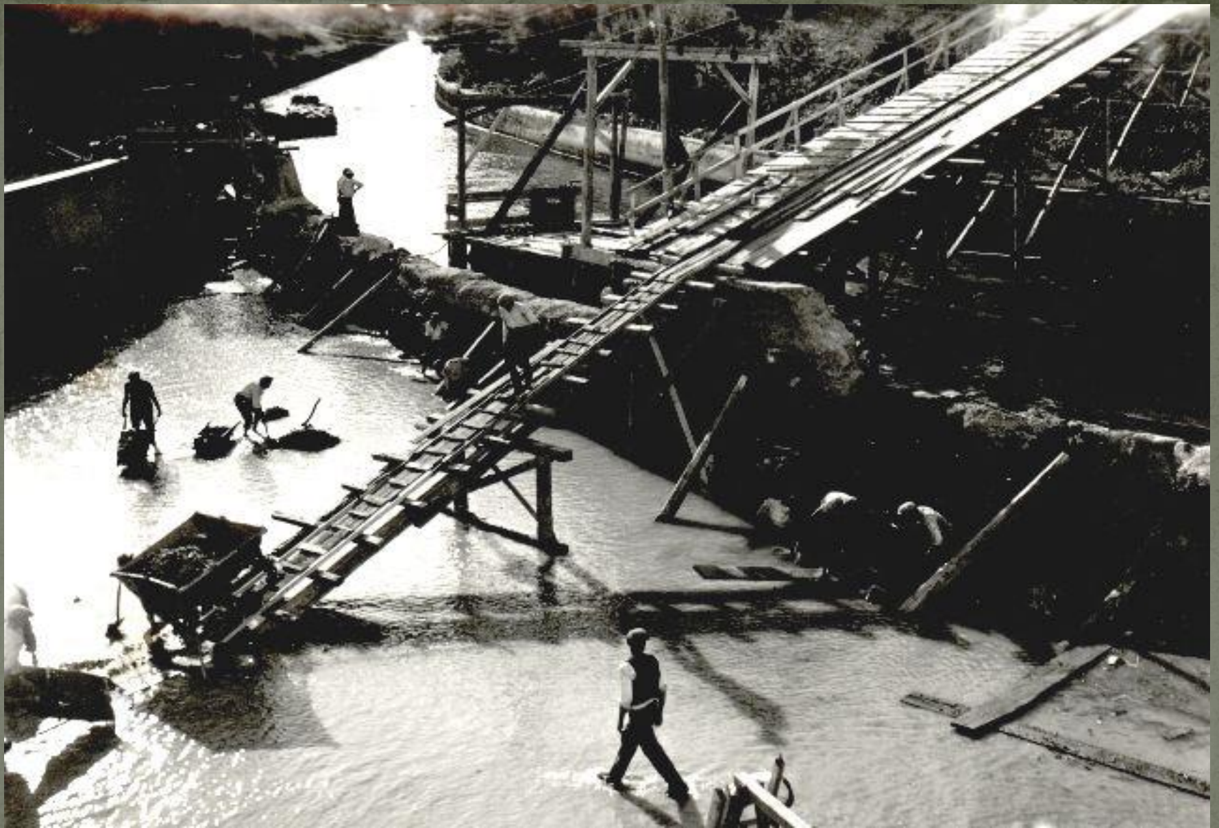
Works in the tailrace canal
