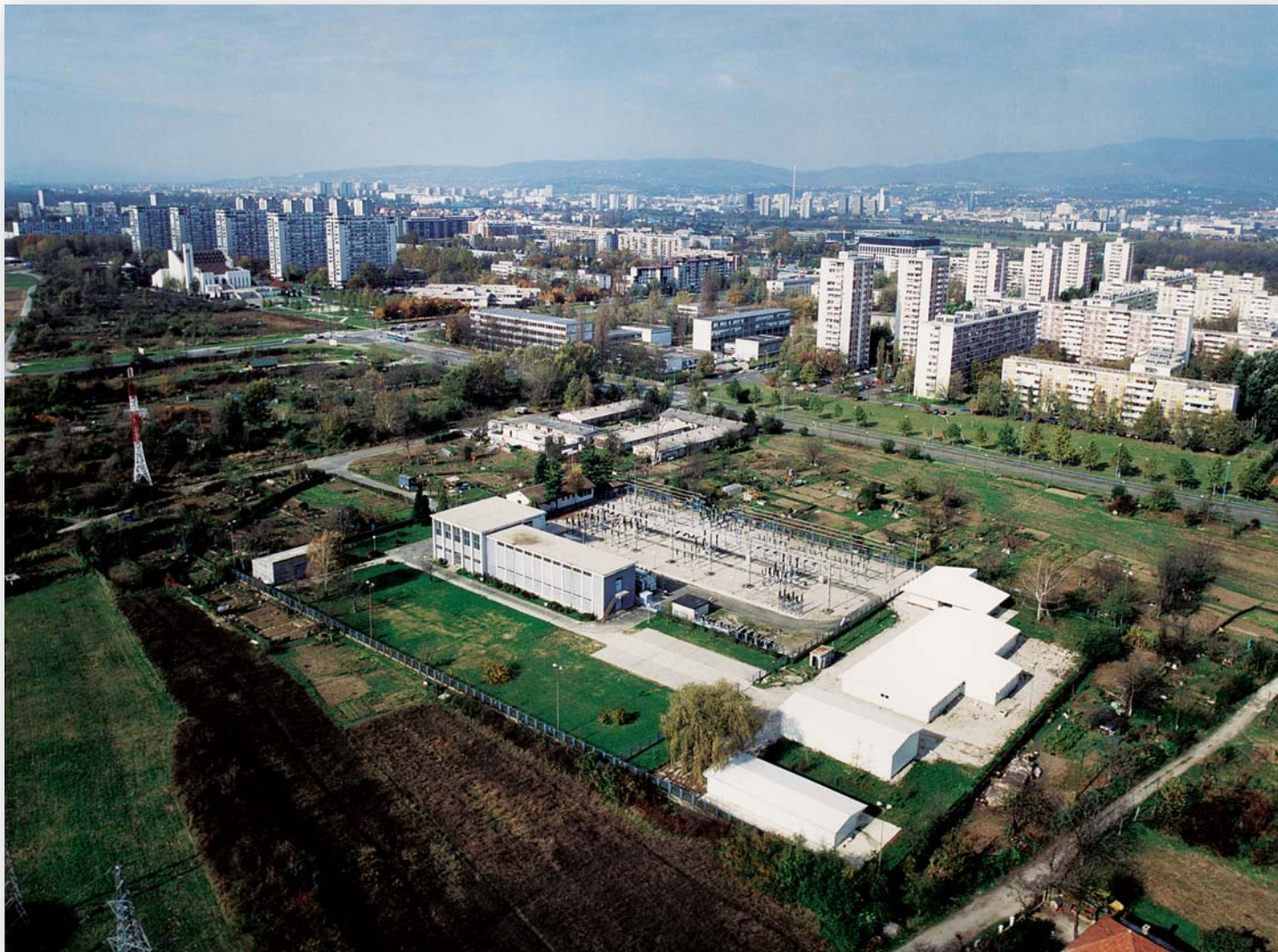
Transformatorska stanica 110/10(20) kV Sopot
