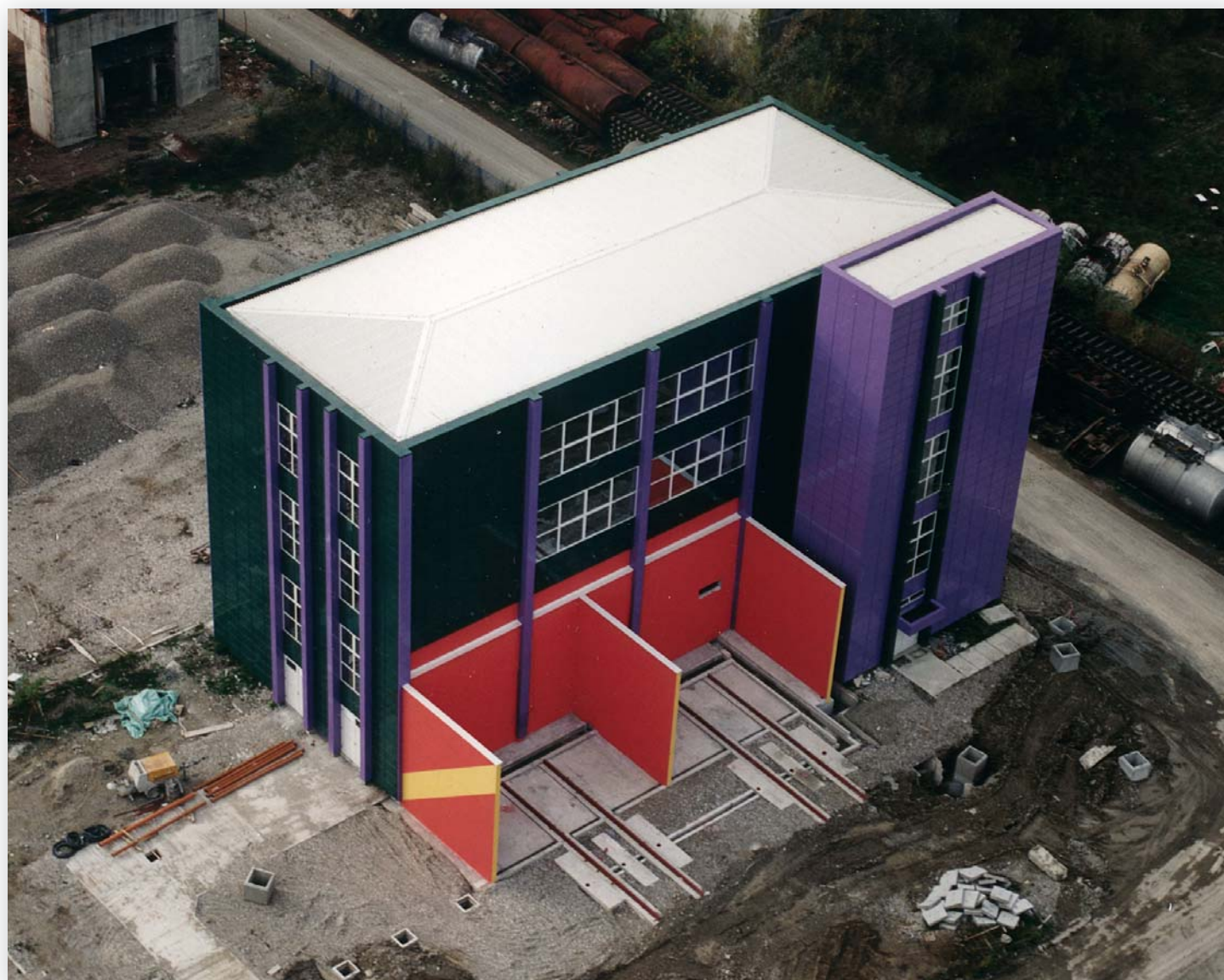
Transformatorska stanica 110/10(20)kV Podsused
