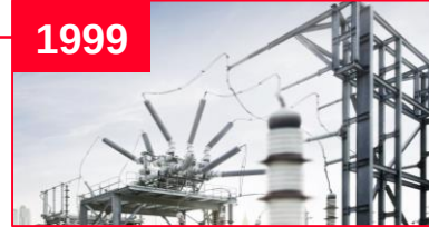
Hybrid switchgear PASS 145 kV
