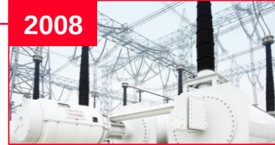
GIS 1100 kV for ultra high-voltage grids
