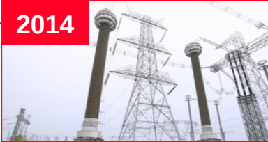
Mixed technology switchgear 1200 kV
