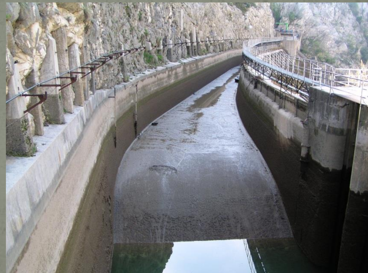
Kraljevac HPP dam
