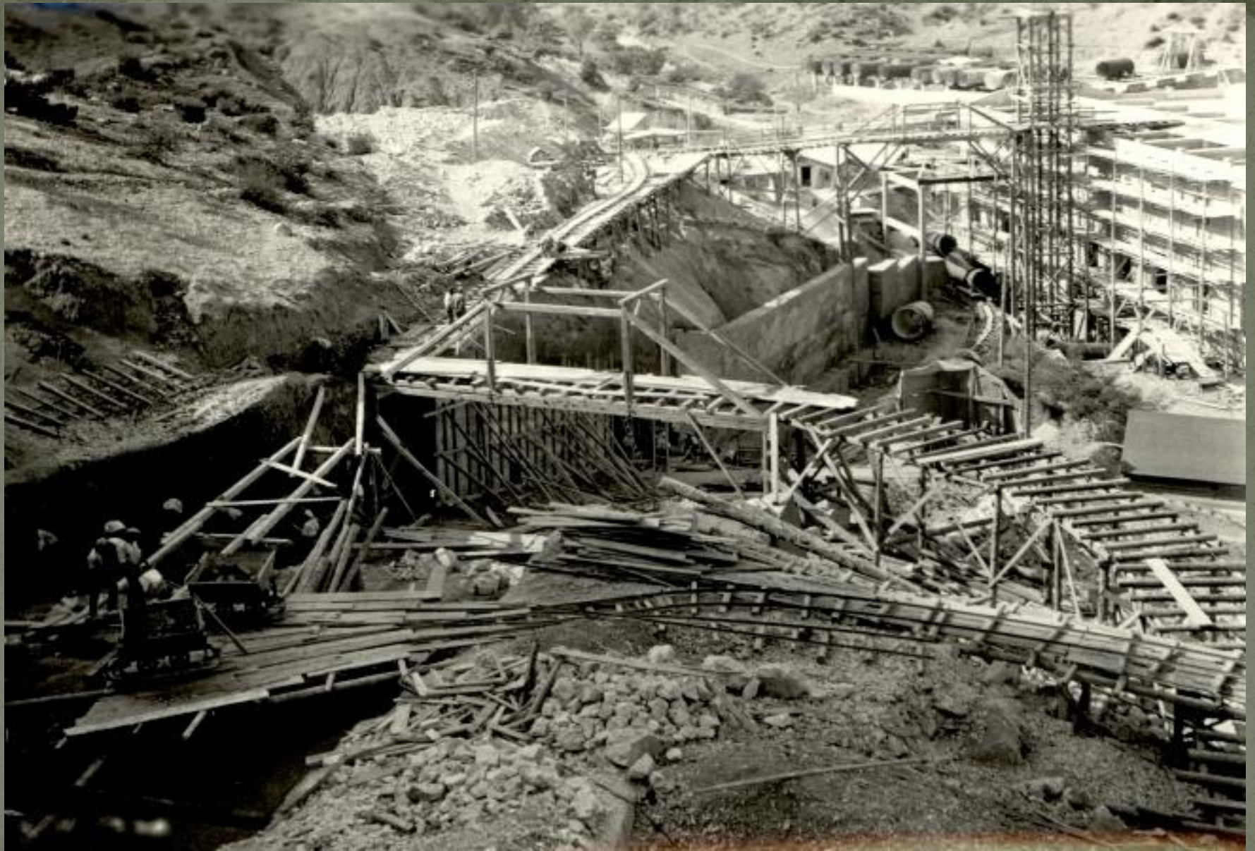
Works on widening the powerhouse and construction of the penstocks 3 and 4
