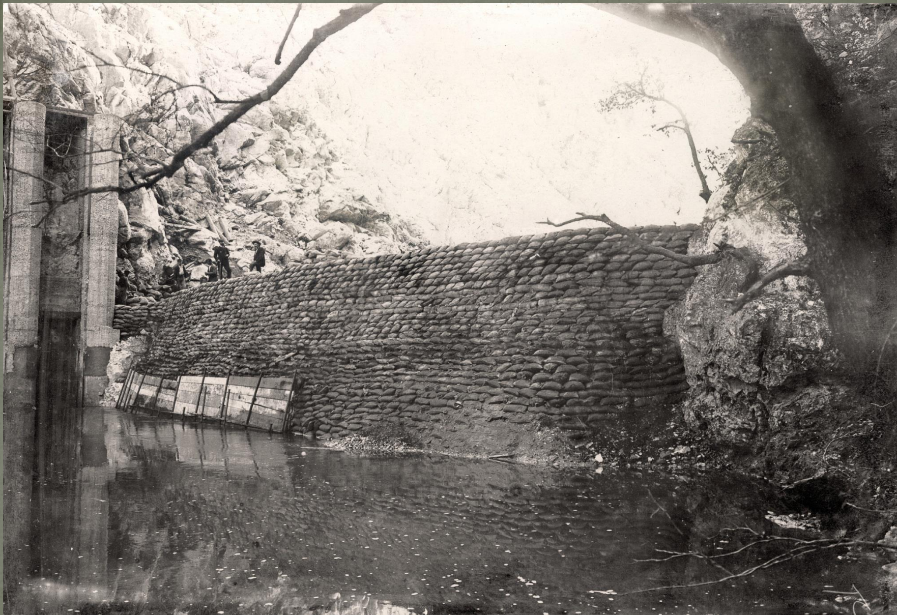
Provisional dam built of 20 000 bags with sand
