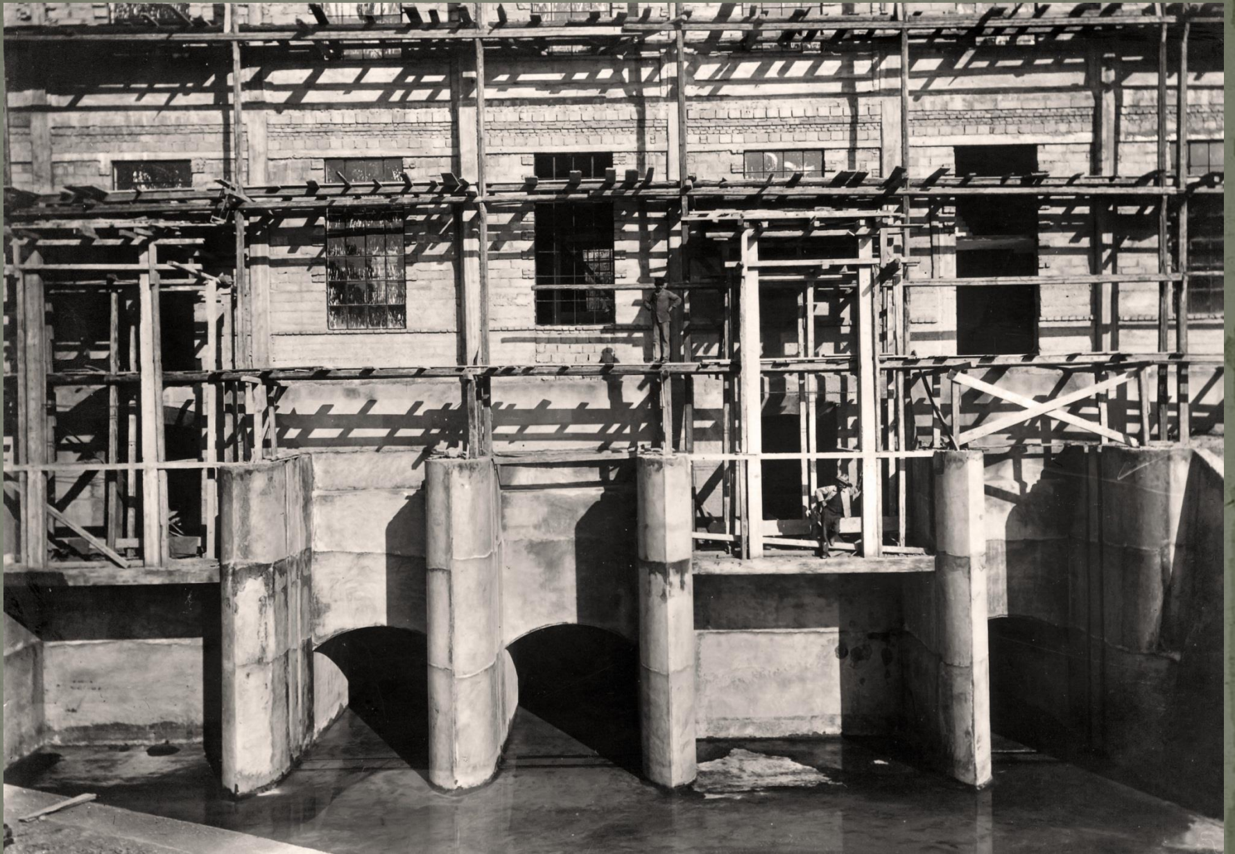
Final construction works of the first stage
