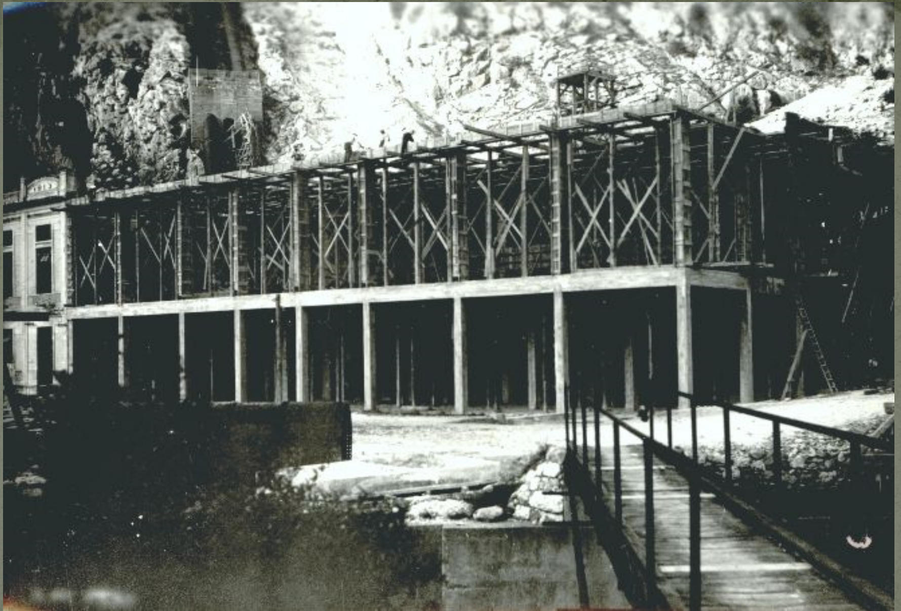
Works of widening the powerhouse are approaching its end
