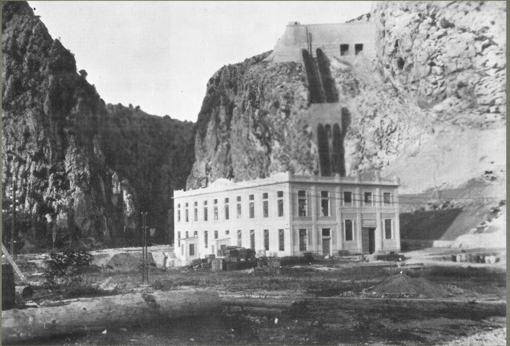
Completed works of the first construction stage
