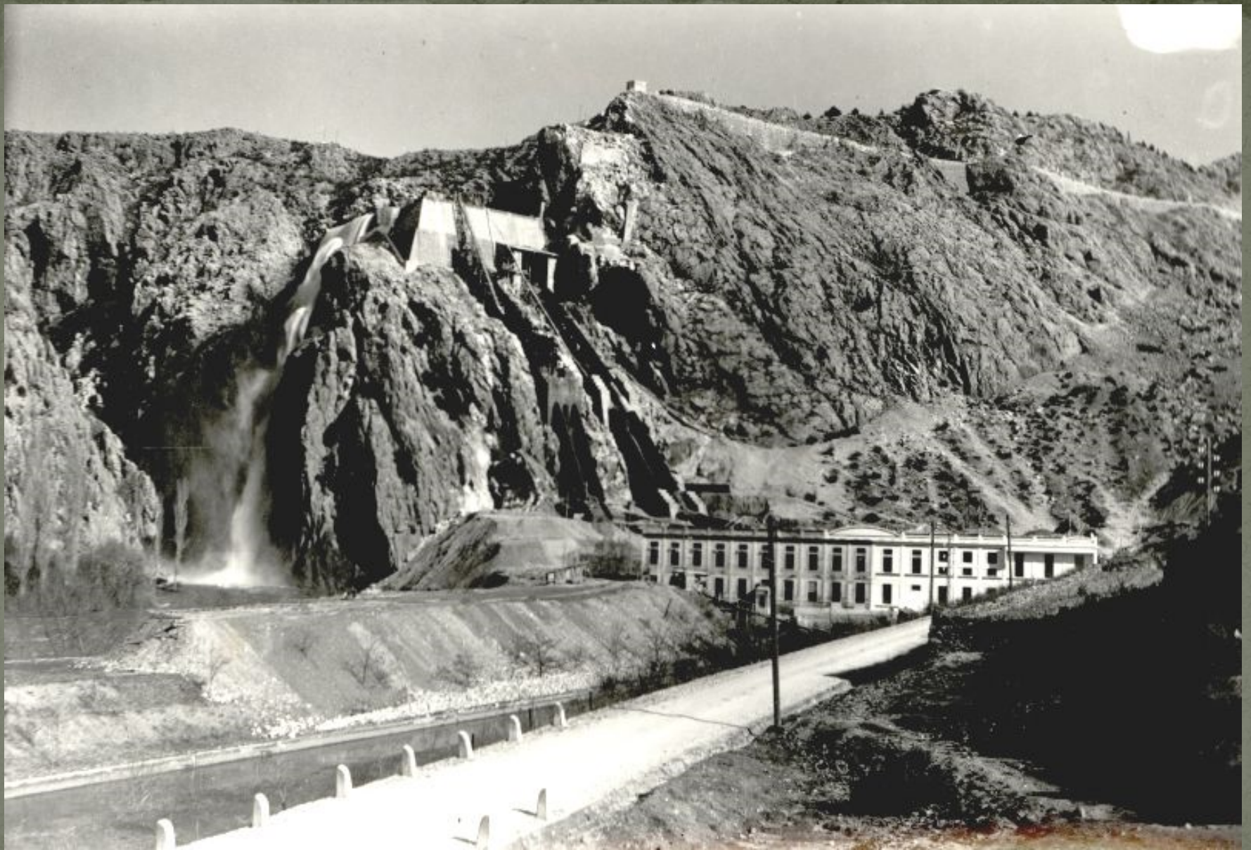
Final works on the second stage (1928 – 1932)
