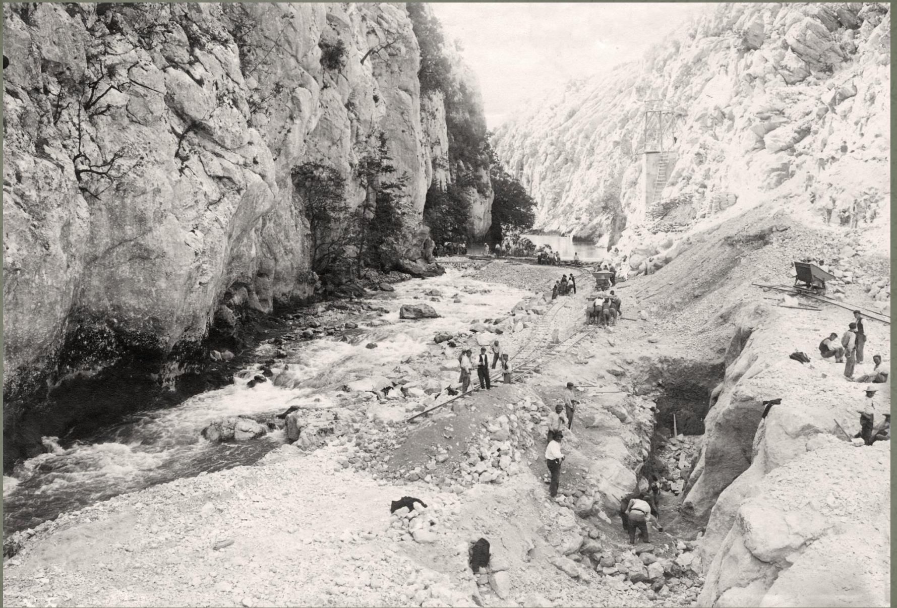
Construction of the dam in 1909
