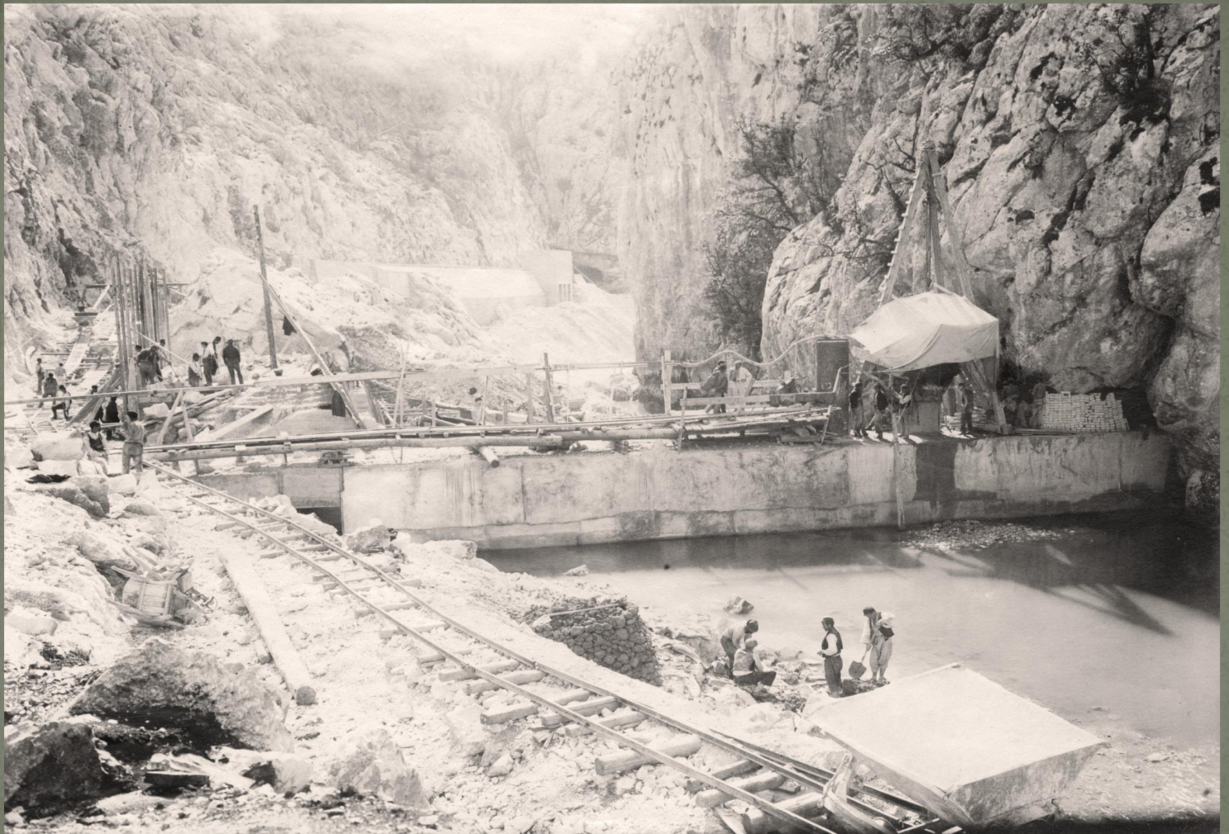
Construction of the dam comes to its end – 1911
