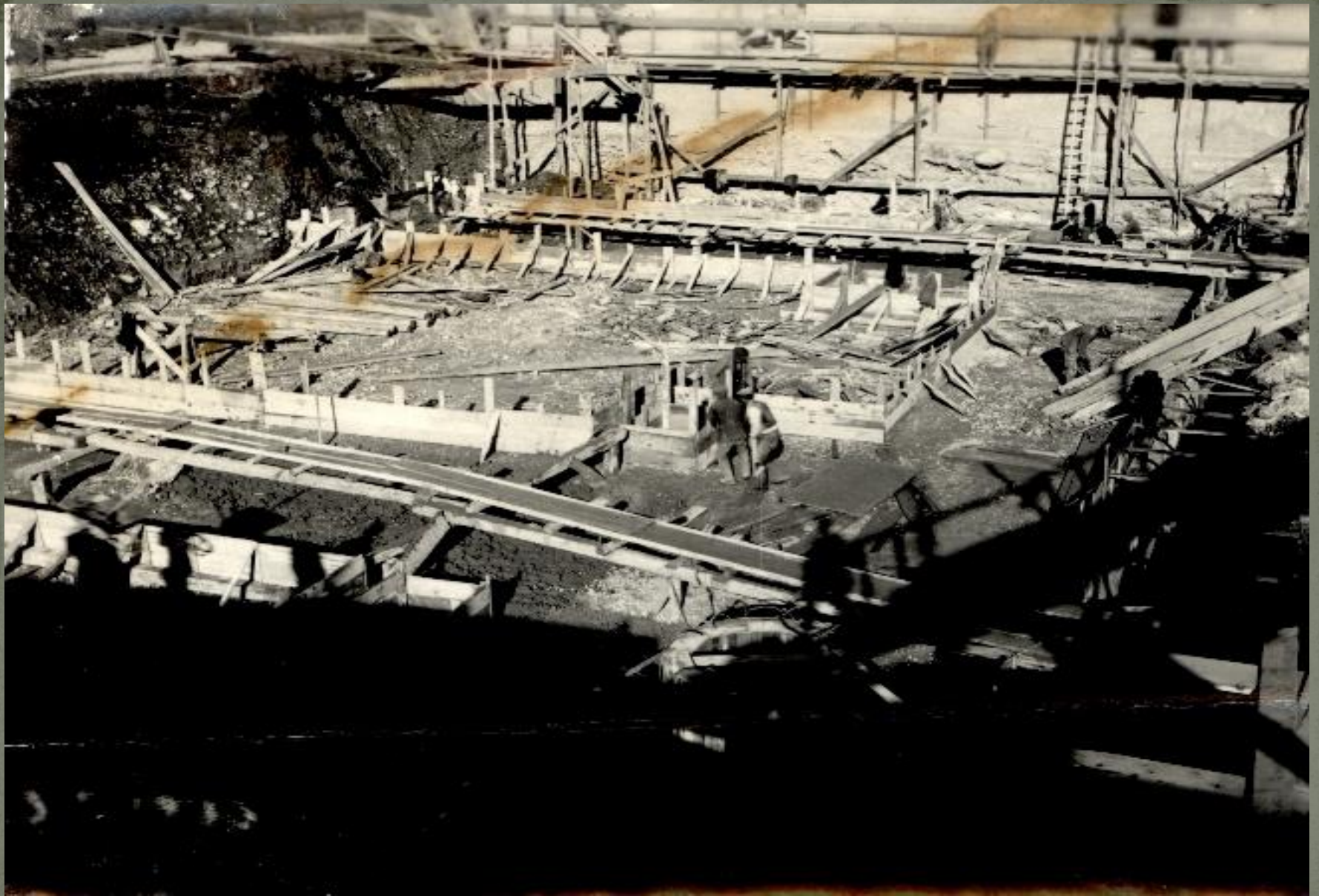
Excavation of the foundations for widening the powerhouse
