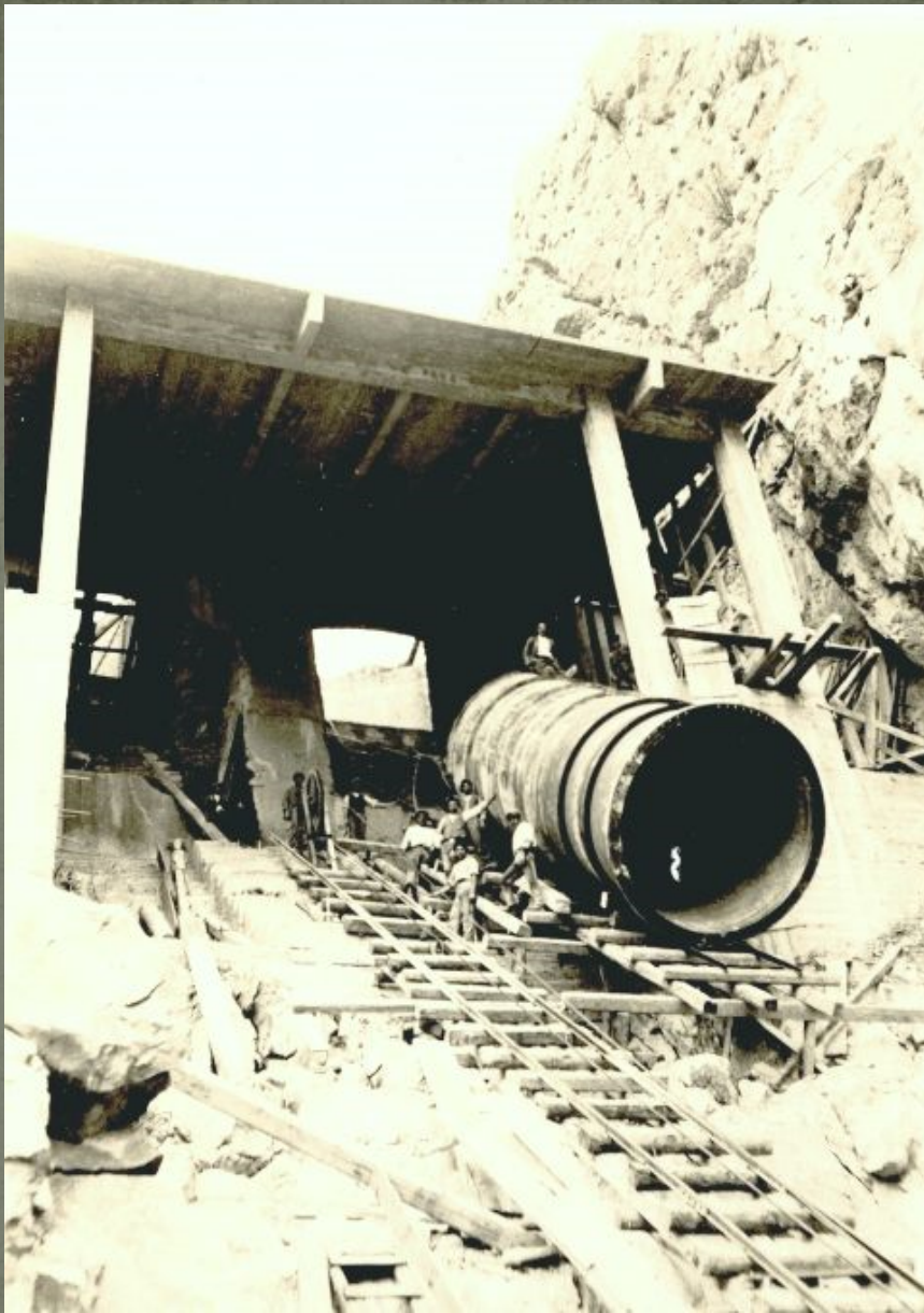
Transportation of the penstock parts to the surge chamber
