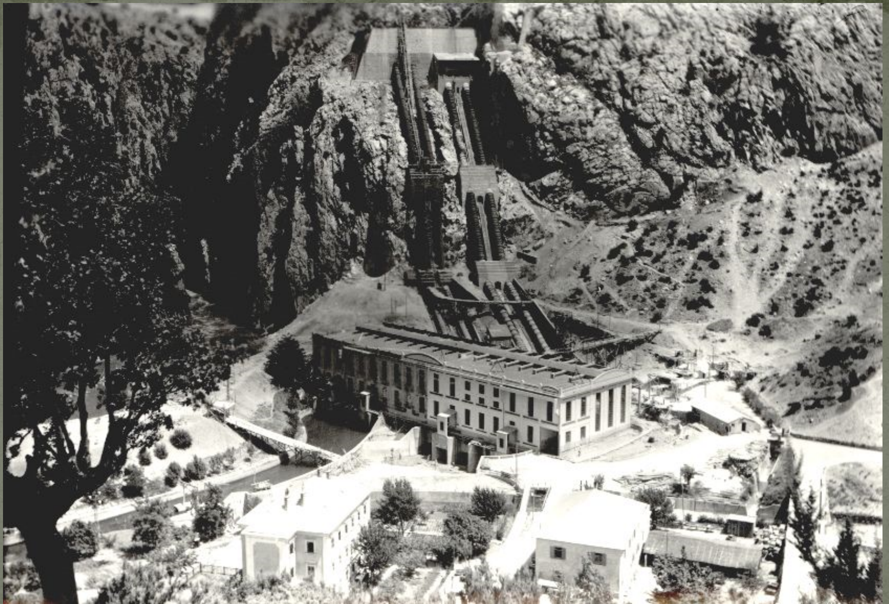
End of the works and demobilization of the site in 1932
