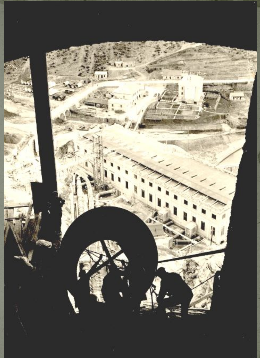
Transportation of the penstock parts to the surge chamber
