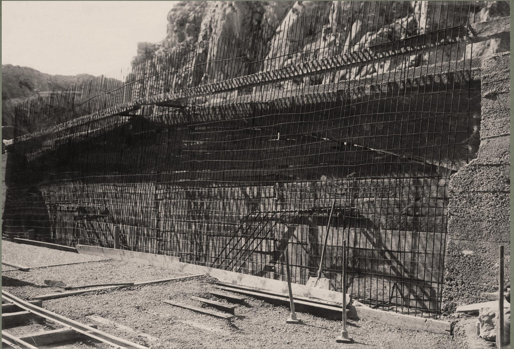
Concrete construction works
