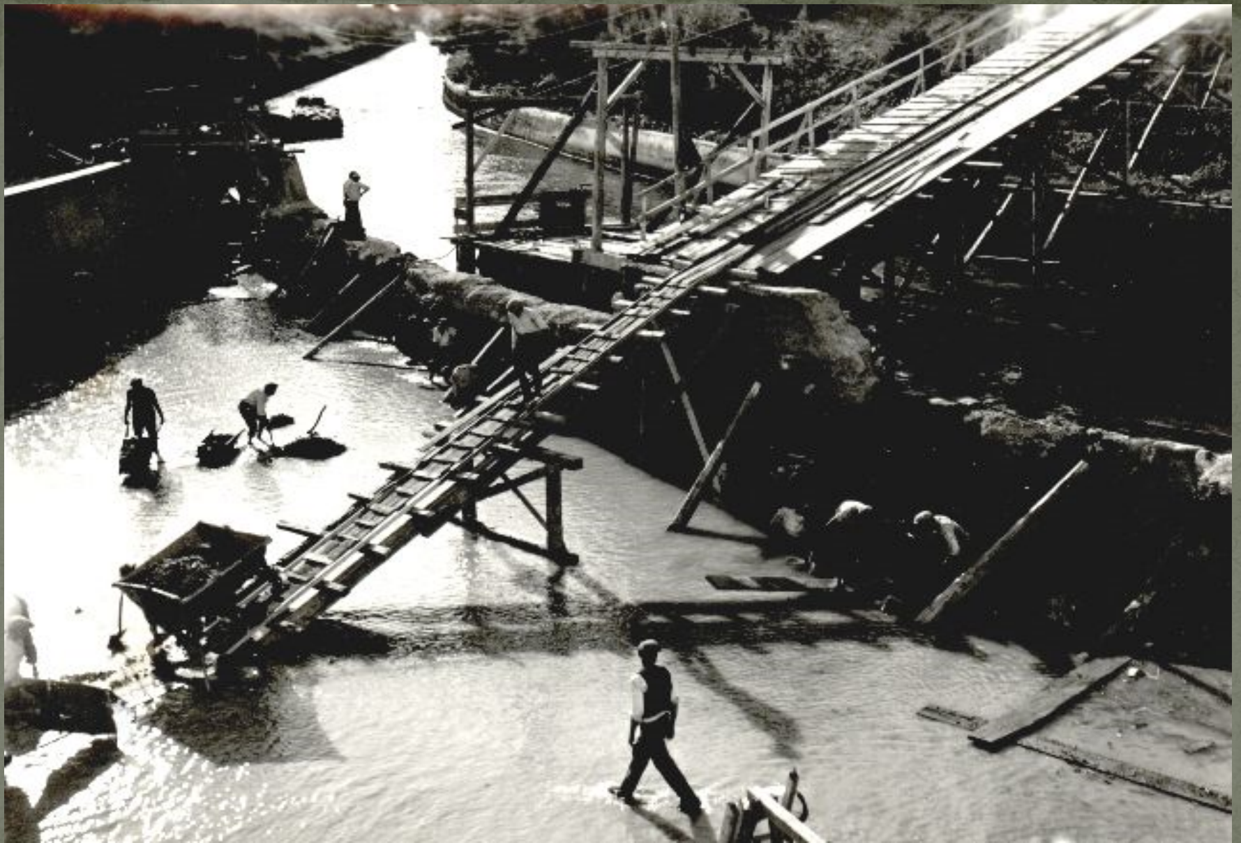
Works in the tailrace canal
