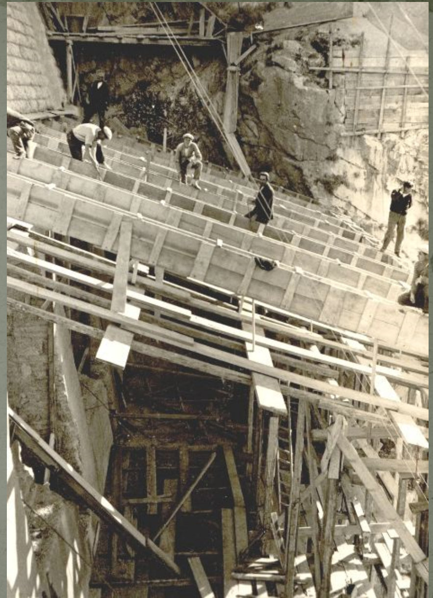
Final works in the valve chamber
