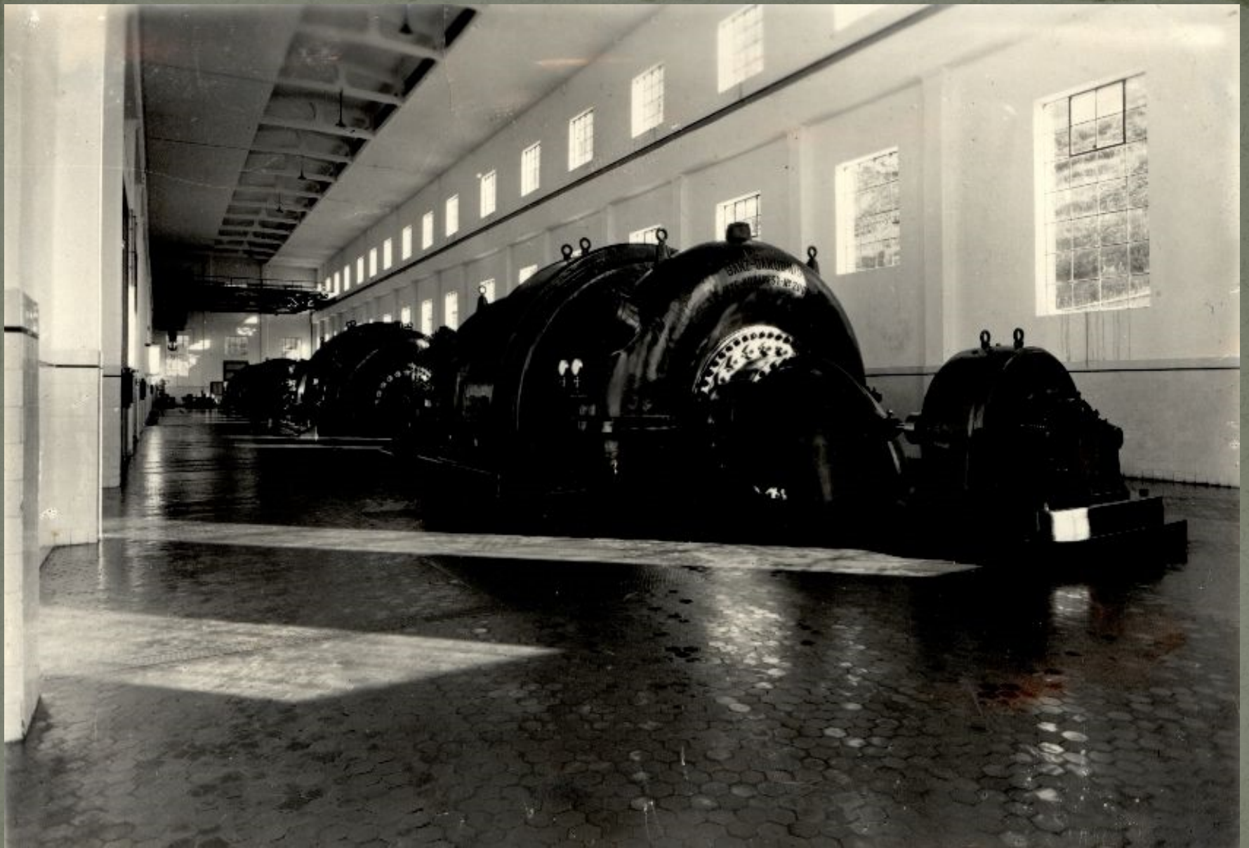
Completed erection works on the generating unit
