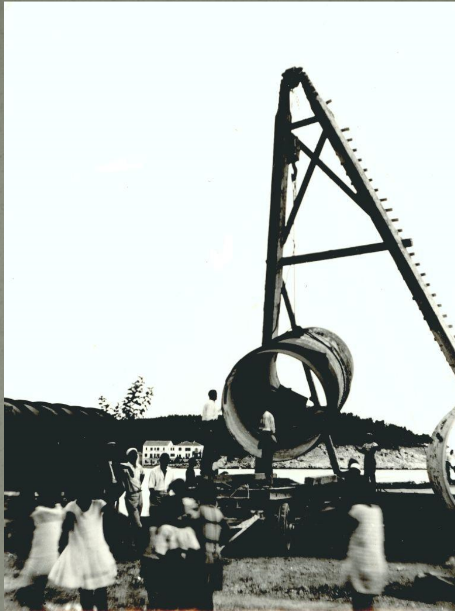
Unloading of the penstocks in Makarska
