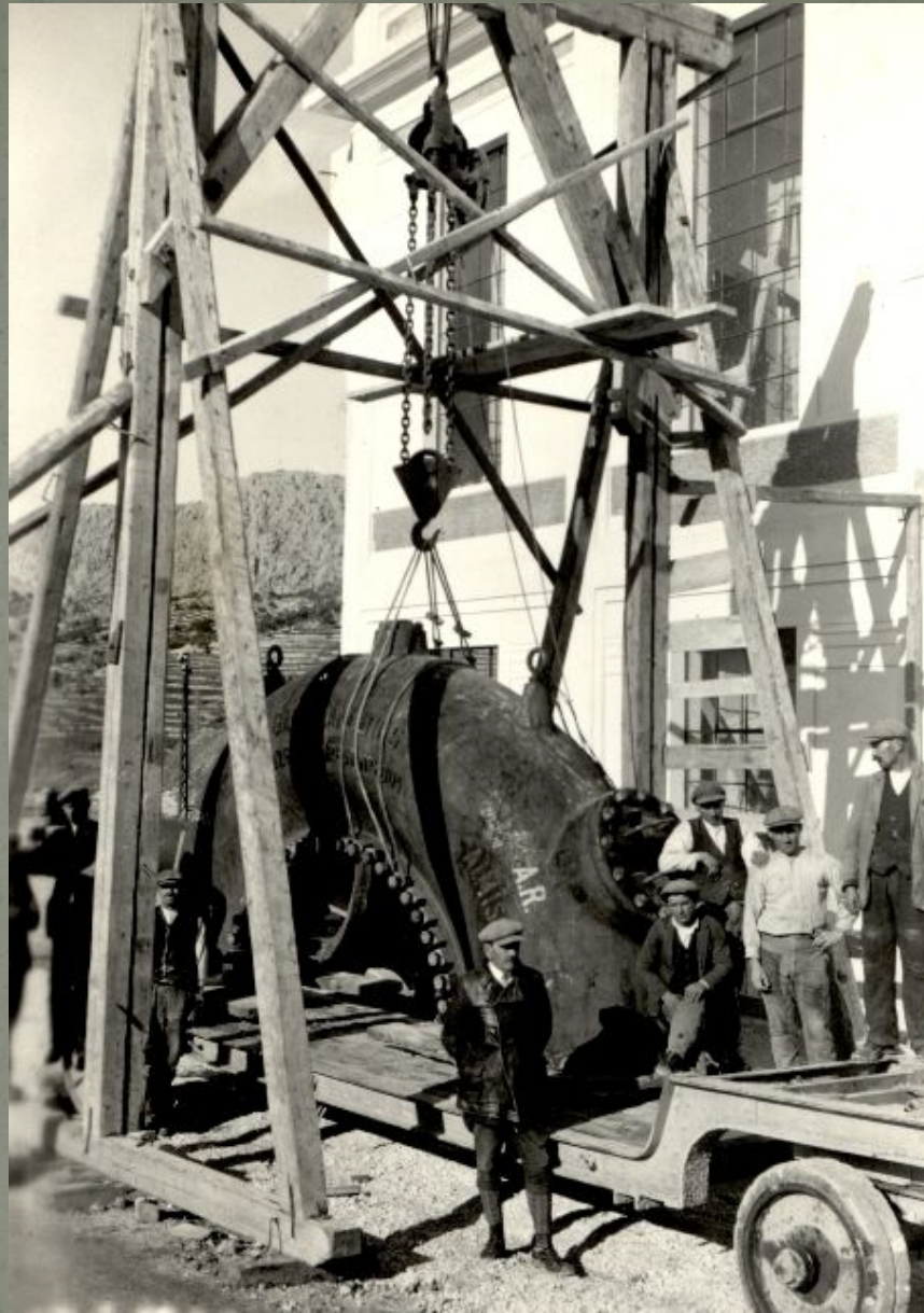
Arrival of the turbine parts on the site
