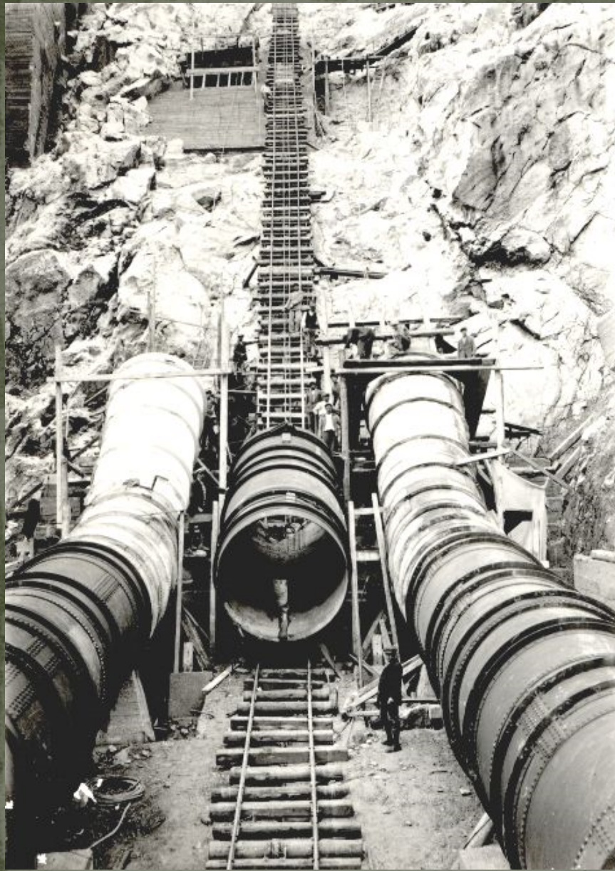
A cable railway for transportation of the penstock parts was constructed
