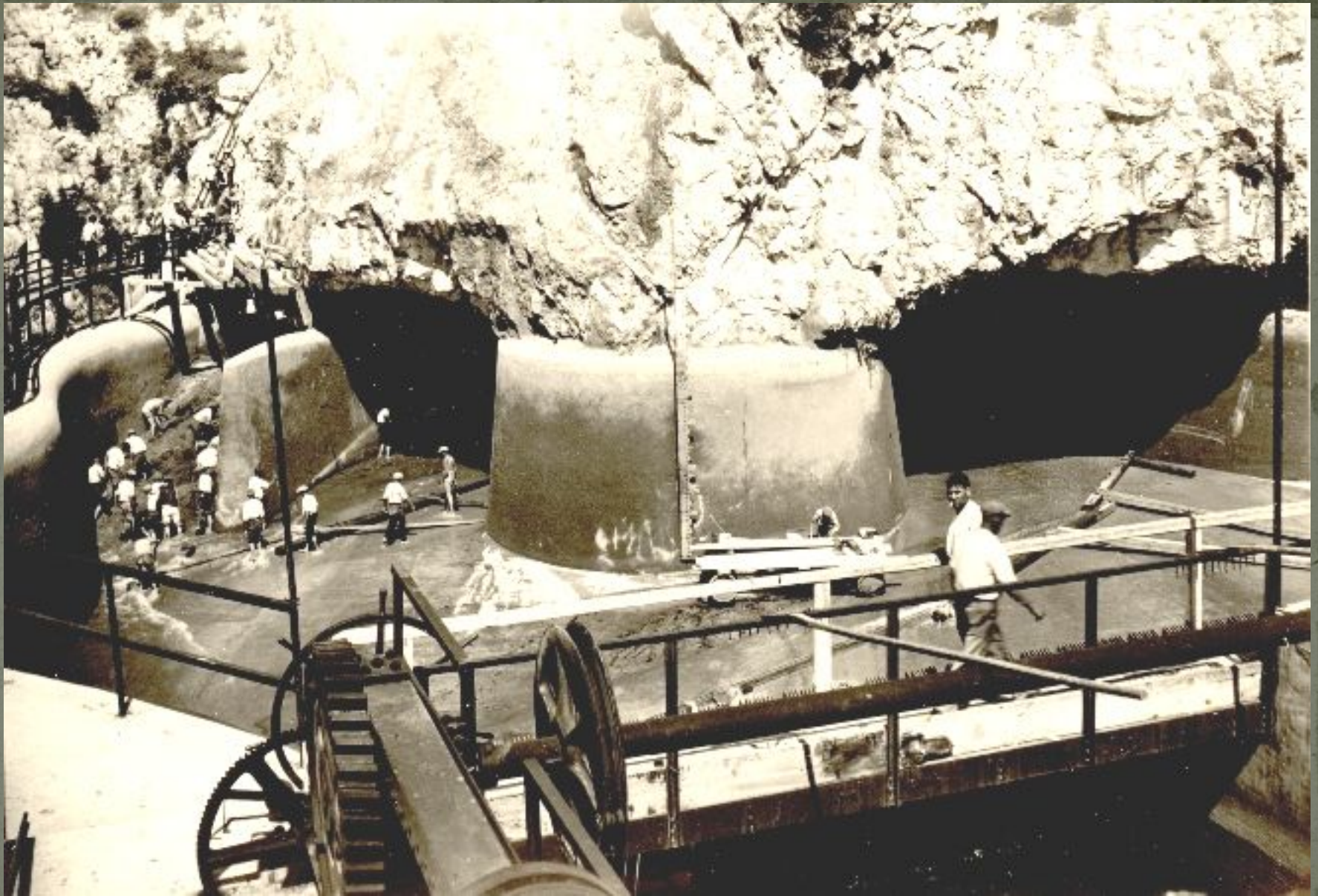
Final works in the surge chamber of the second stage
