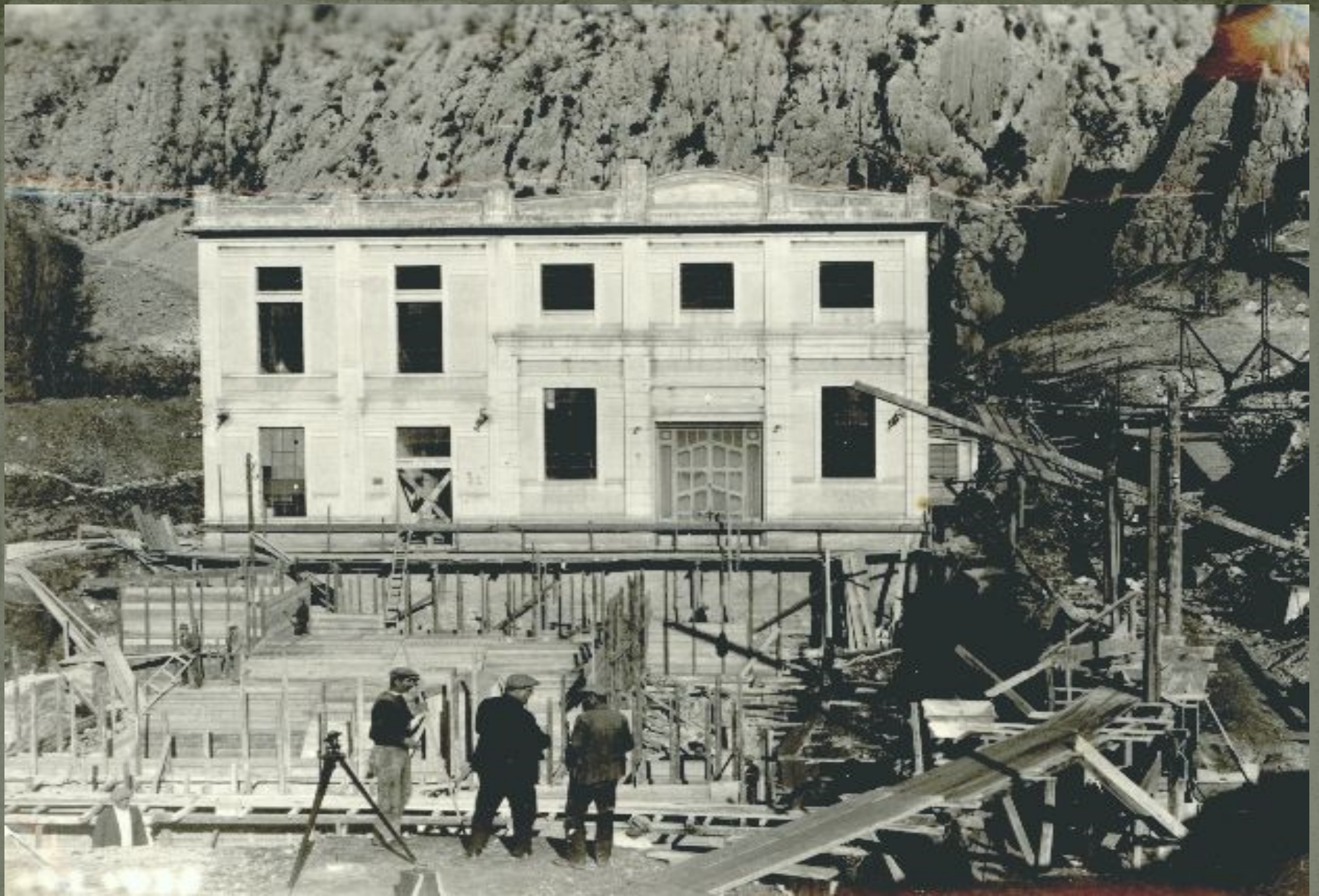
Works on widening the powerhouse
