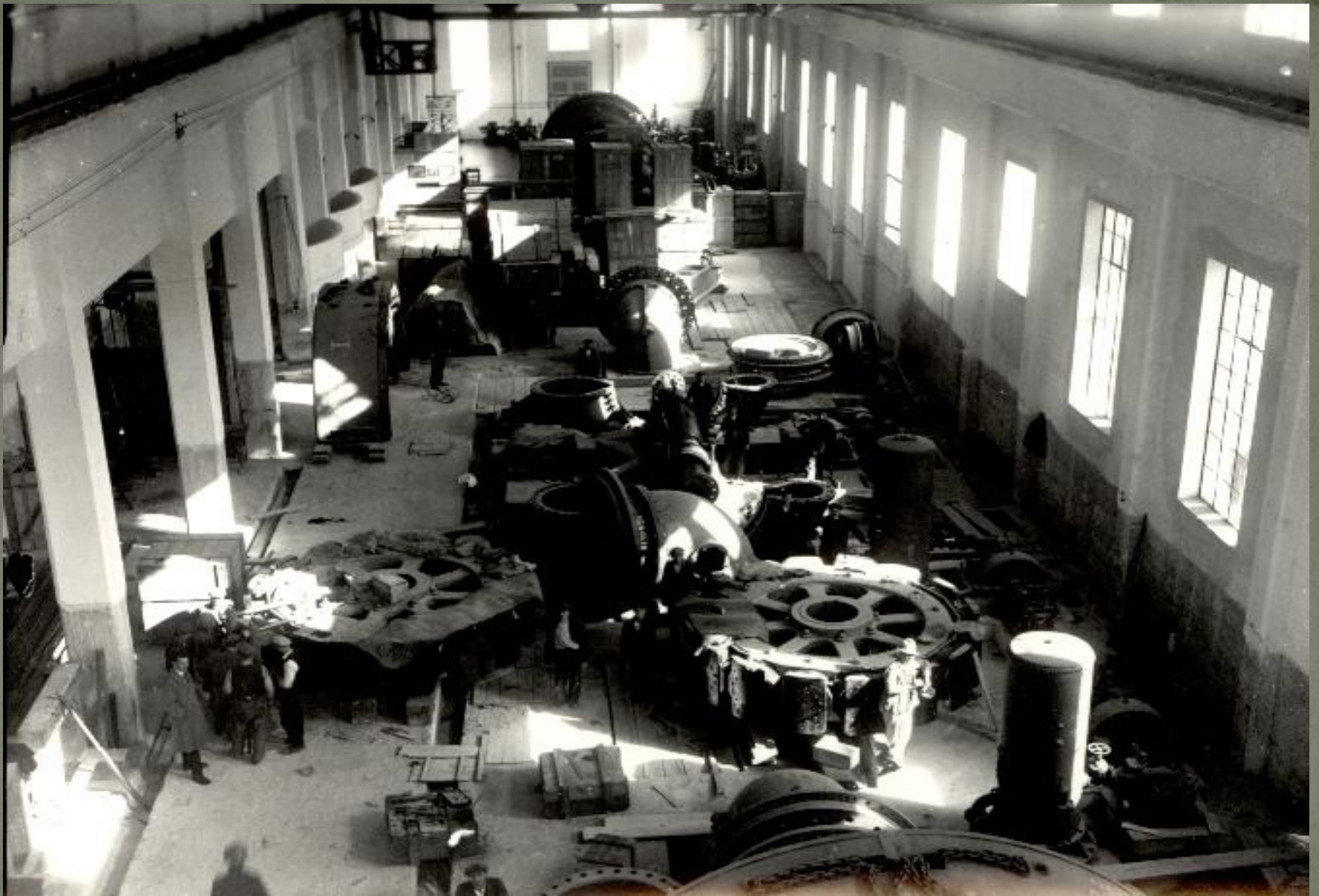
View of the powerhouse
