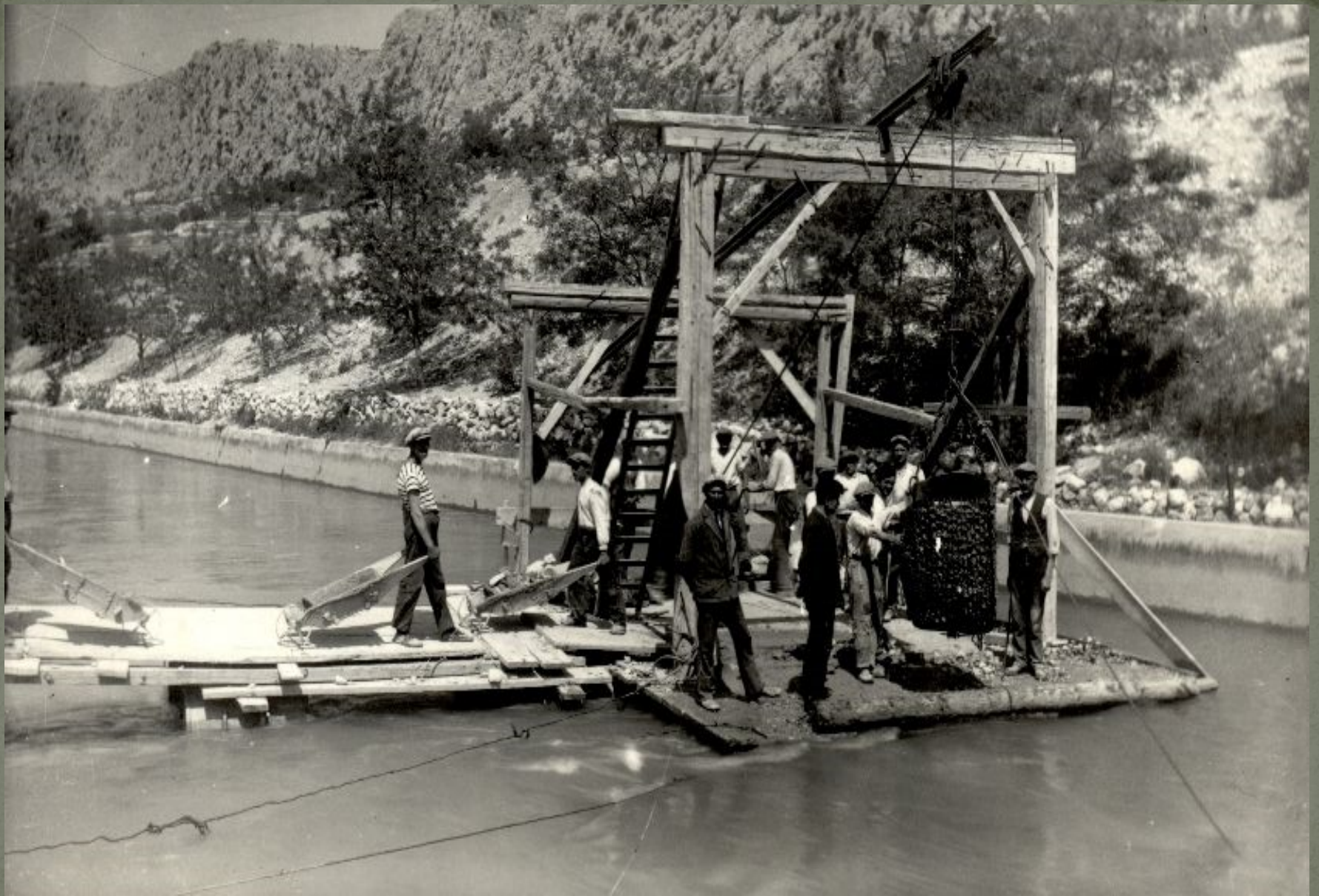
Works in the tailrace canal
