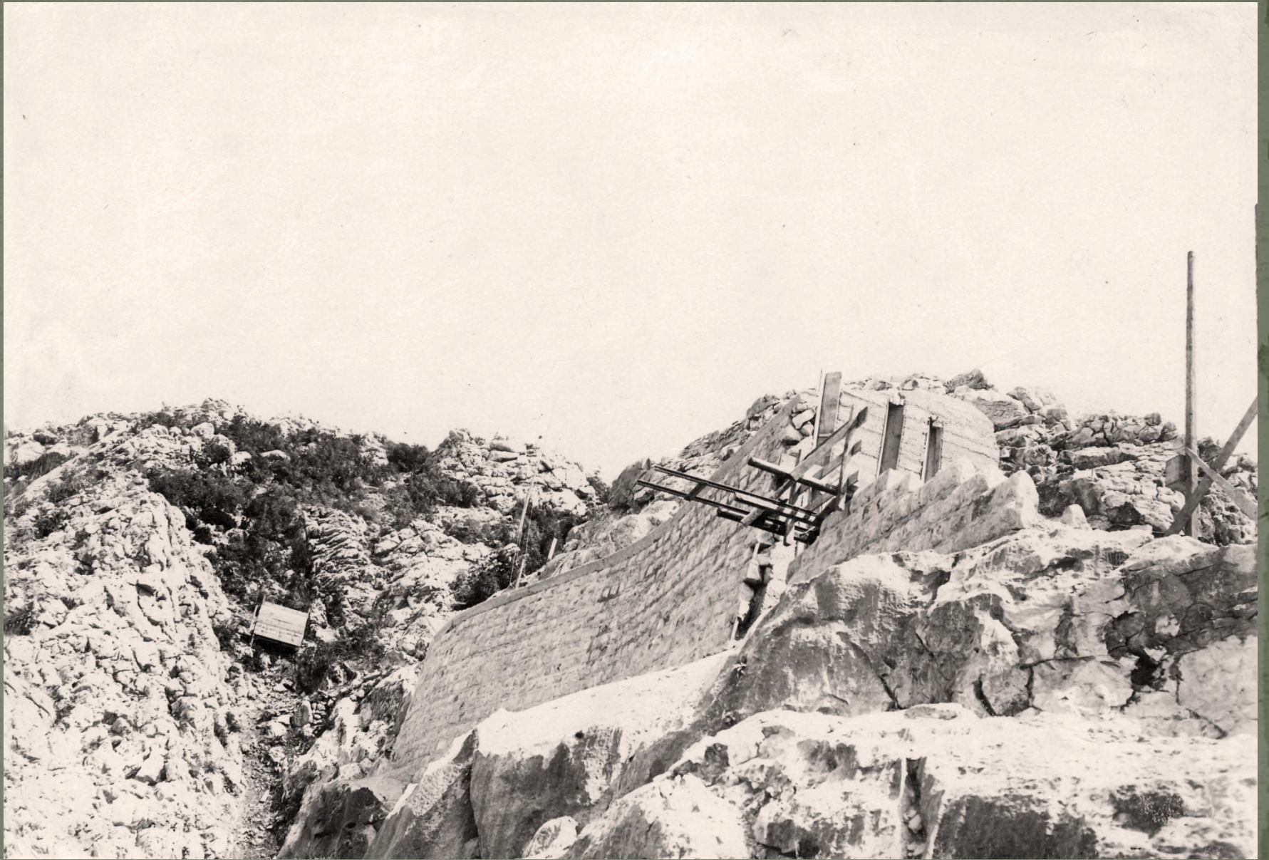
Construction of the surge chamber spillway wall
