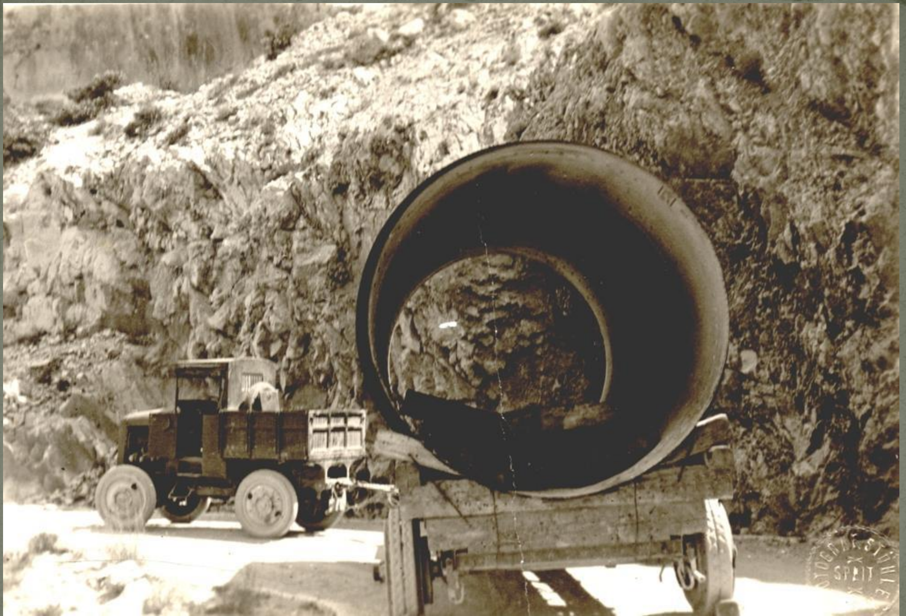
Transportation of the penstocks Makarska - Kraljevac
