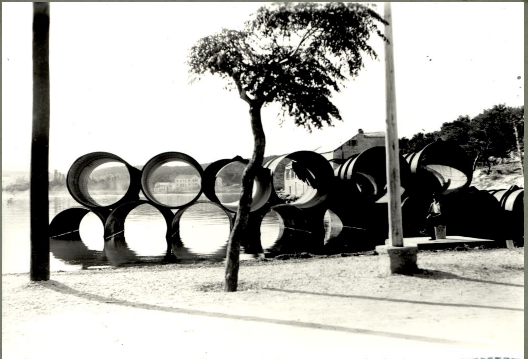
Parts of the penstocks on the Makarska beach
