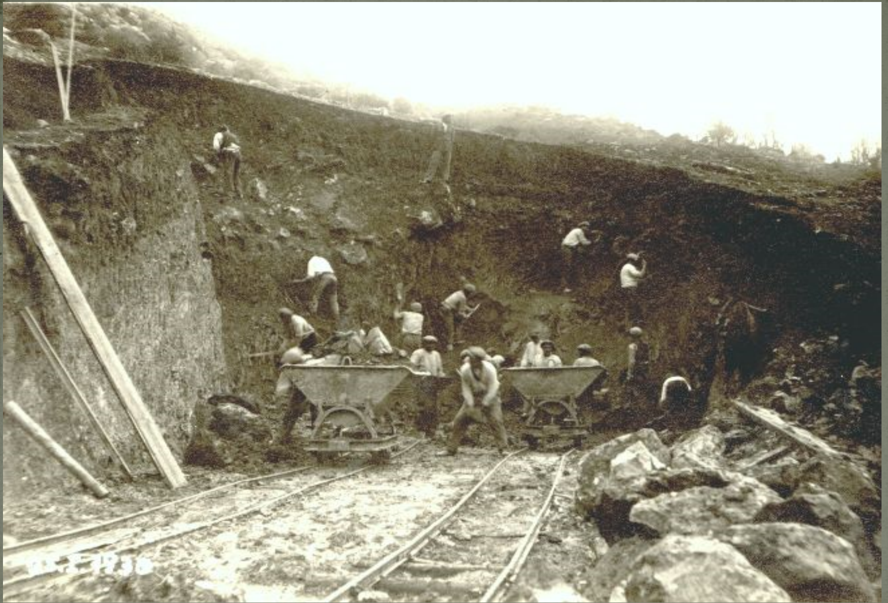
A great number of workers took part in construction works
