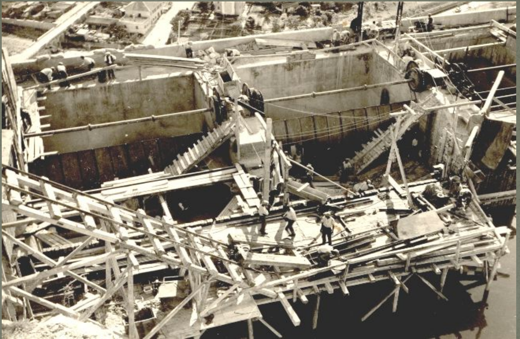
Final works in the surge chamber of the second stage
