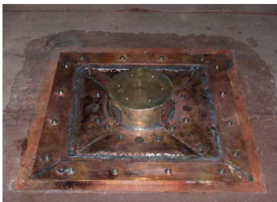
Figure 3. Earth plate electrode
