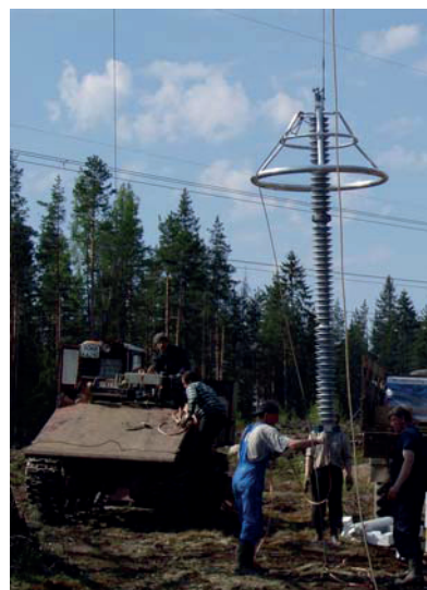
Figure 4. Installation of LSA
