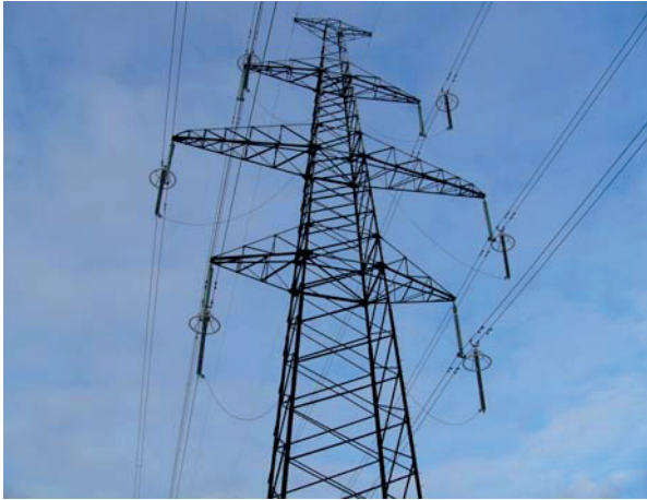
Figure 5. “Trouble tower” with arresters. installed in both circuits and in all 6 phases.
