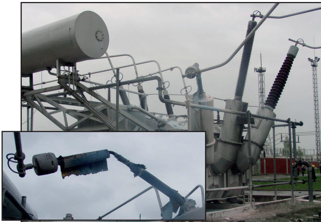
Figure 9: Bushing terminal failure in 2003 and traces of fire on the 300 MVA, 400 kV autotransformer; The right-hand bushing in the figure was replaced after an incipient failure in 1994. Detail shows the bushing debris and the tubular connection dilatation compensator
