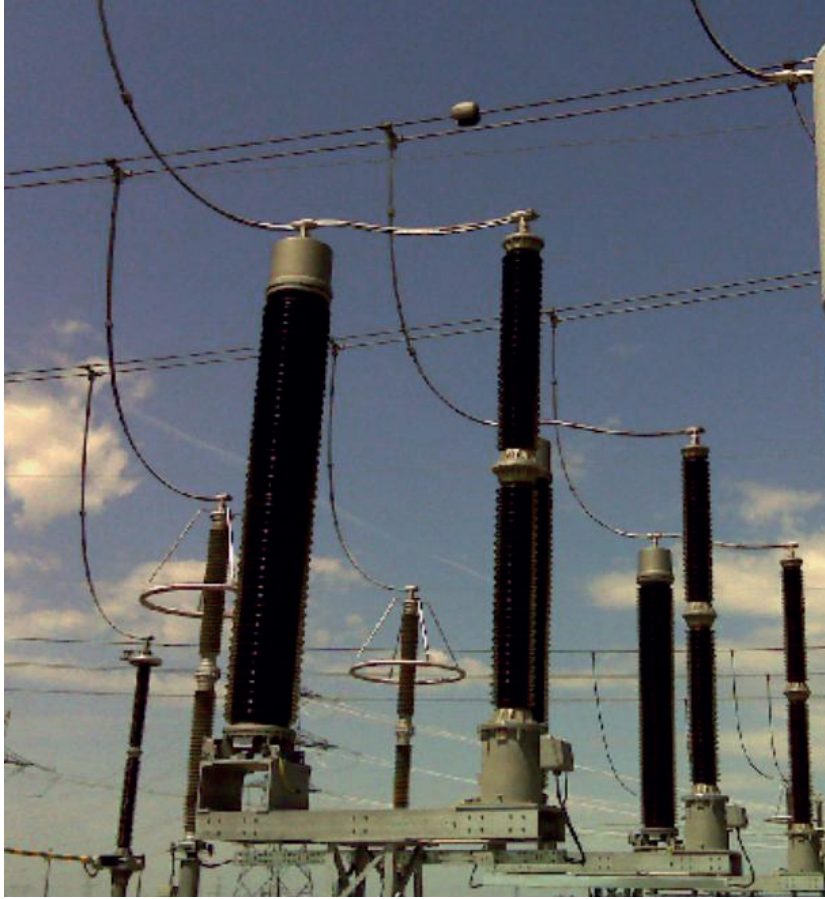
Figure 1 – Simultaneous work of capacitor and inductive voltage transformers in a 400/110 kV substation
