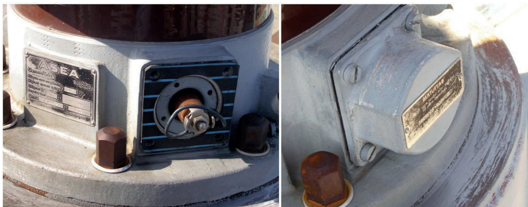
Figure 17 – Measuring tap on ASEA bushing from 1965.
