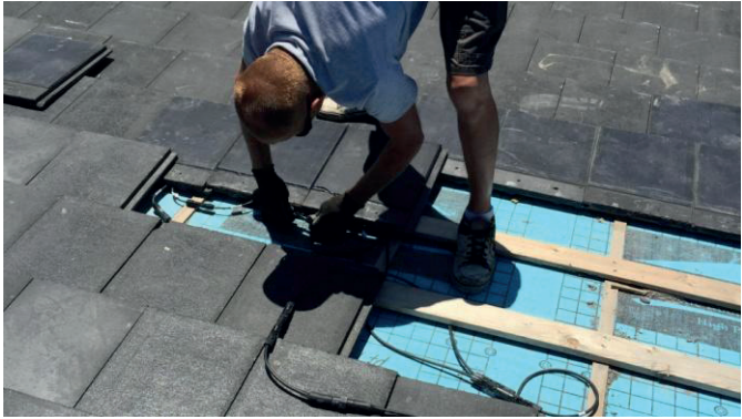
Figure 3. An integrated solar cell in roofing, [4]
