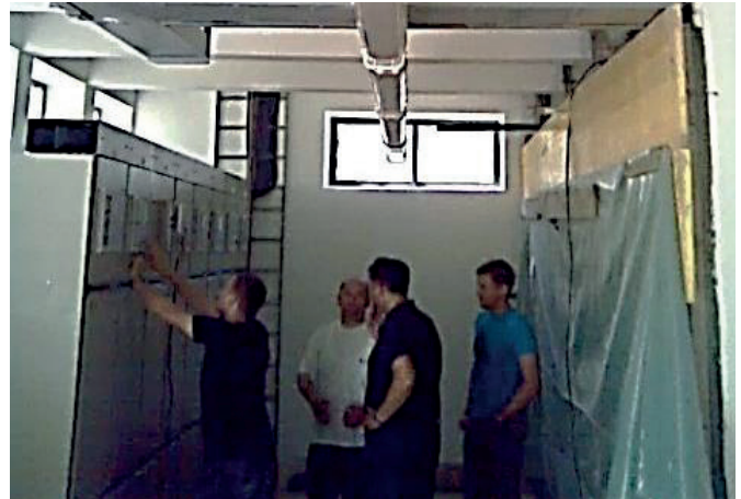
Image 7 Works on the new 10(20) kV plant
