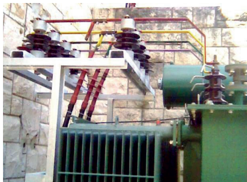
Image 9 Bracket of support insulators, surge arresters and cable terminals on a 10 (20) kV side of the power transformer
