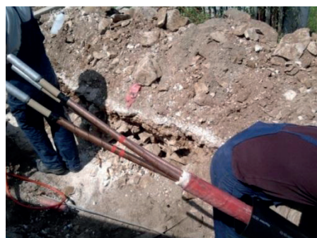
Image 13 Making of cable joint
