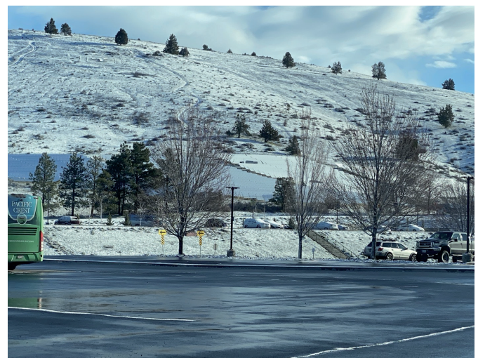
Fig. 1. Solar panel arrays covered with snow.
