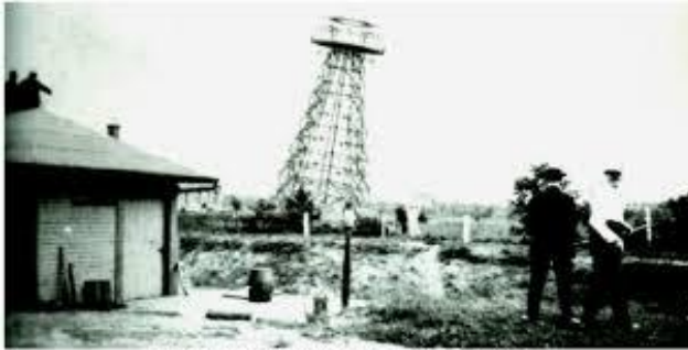
Tesla tower being torn down July 4, 1917
