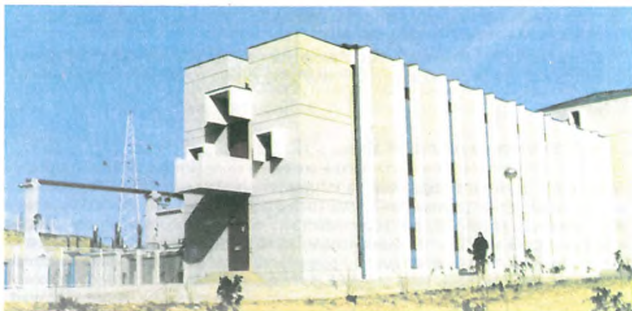
Sl. 8. 23. TRANSFORMATORSKA STANICA SPLIT III, 110/10 kV (1982. g.)
