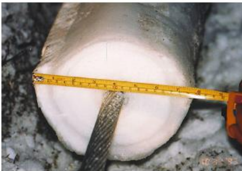
Figure 4: Wet snow accretion on overhead conductor
