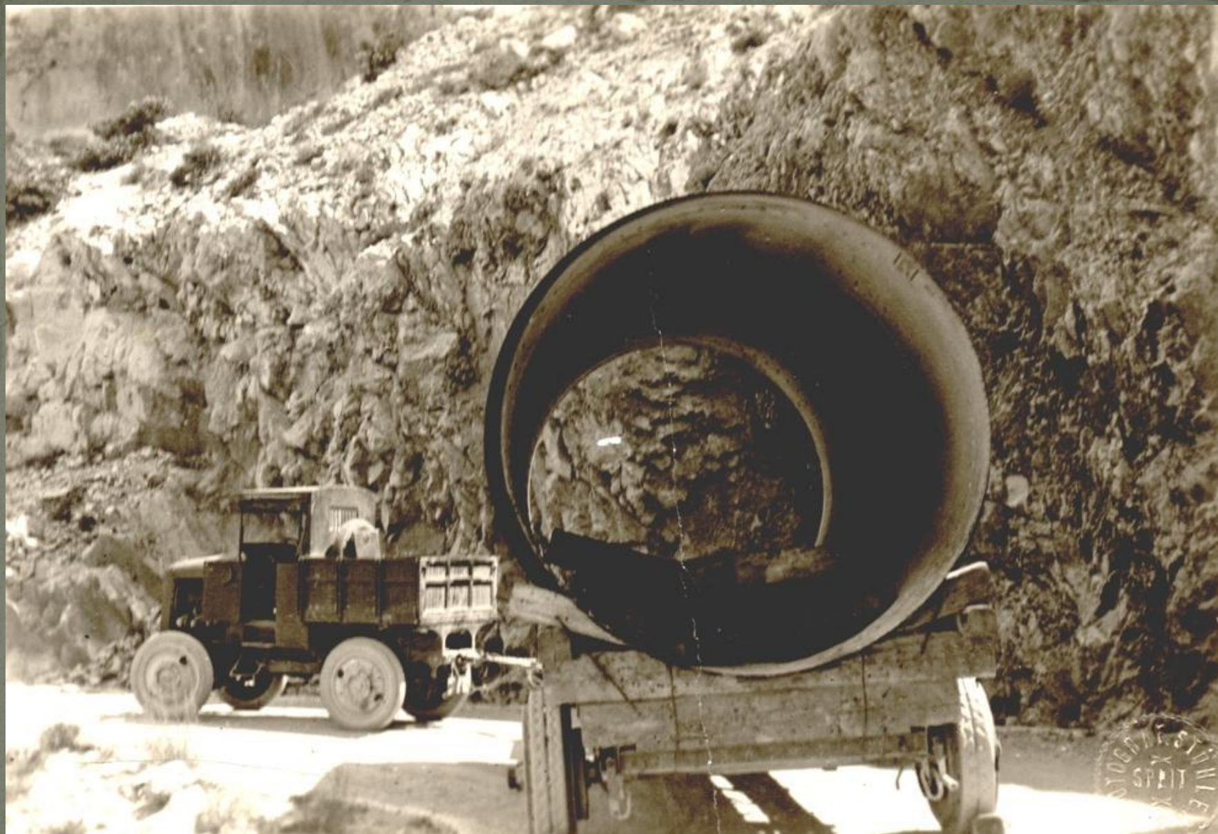
Transport cjevovoda Makarska - Kraljevac
