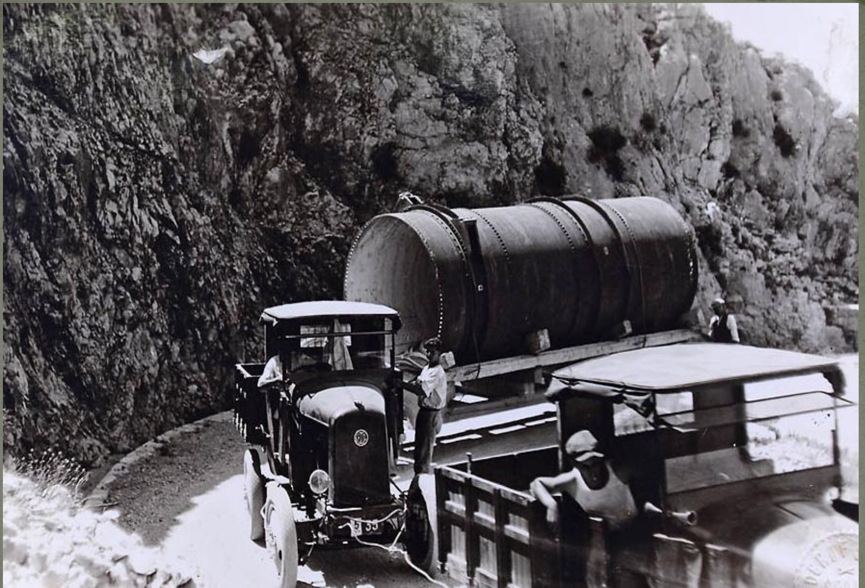
Transport cjevovoda Makarska - Kraljevac
