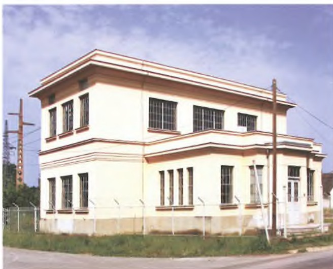
Transformatorska stanica 35/10 kV Ilovac
