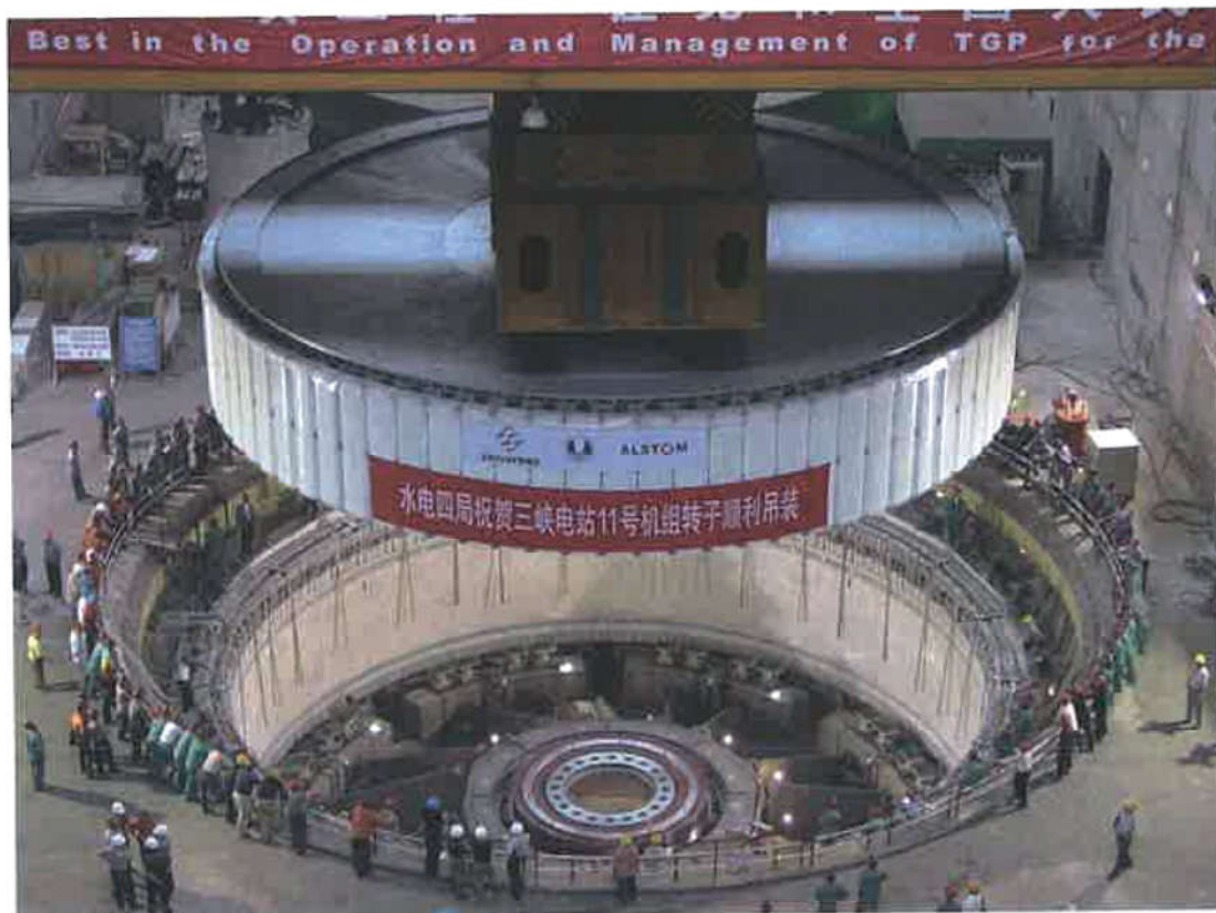
Fig. 2: One of the 84-pole 700 MW/20 kV hydro generators for the Three Gorges power station in China in 2003 while the rotor was being inserted in the stator bore. (Source: ALSTOM Power Hydro)
