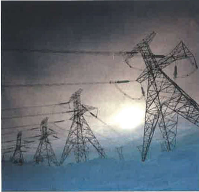
[735-kV angle towers at James Bay, Québec]
