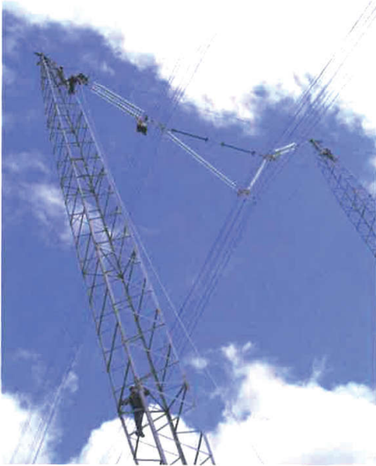
500 kV high surge impedance loading (hsil) line experimental prototype monitored in Rio de Janeiro
