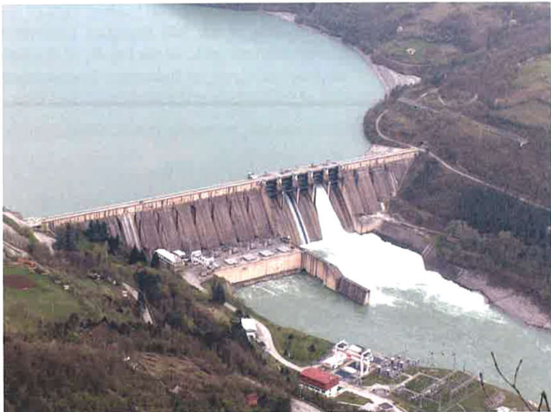
Run-of-River and pumped storage HPP Bajina Basta Serbia
